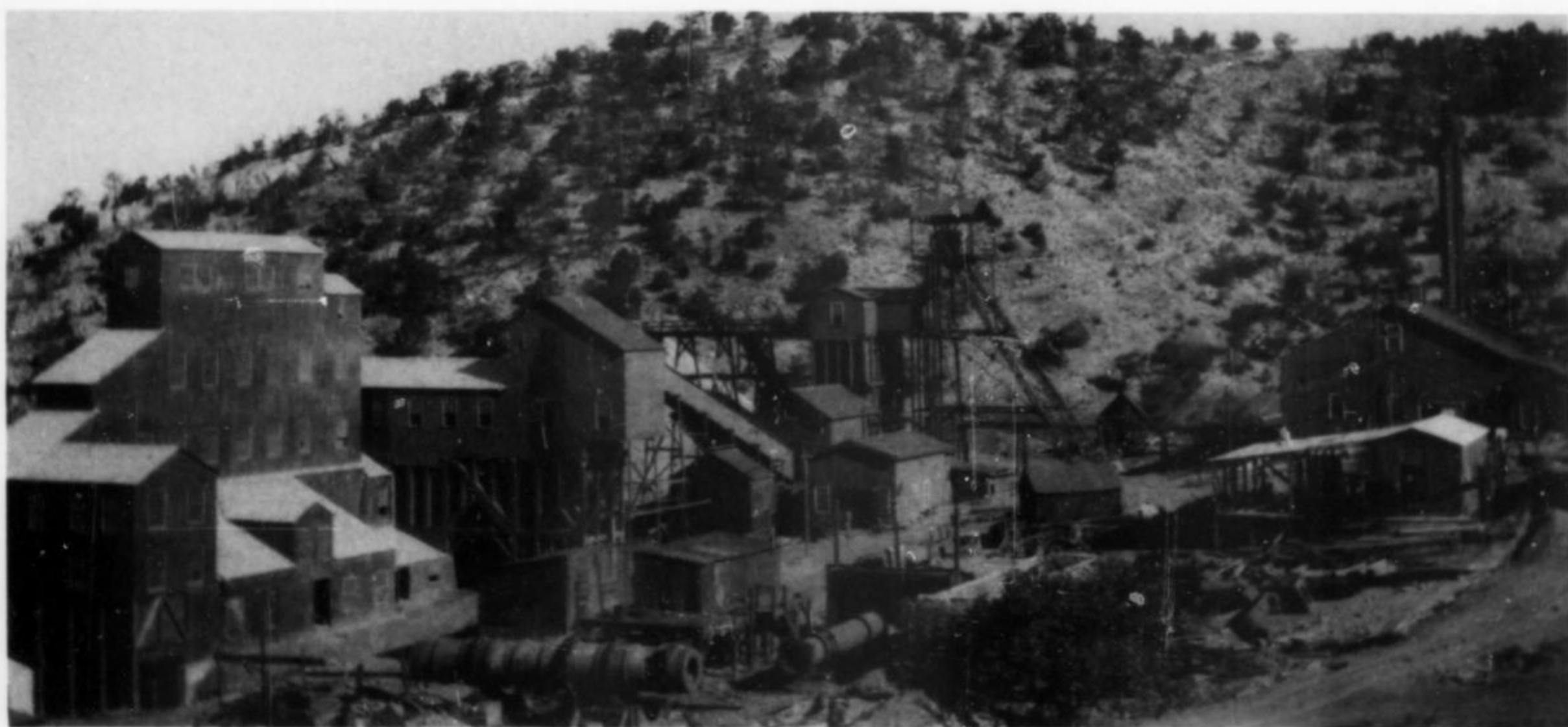
Figure 1. The Kelly mine, surface facilities, ca. 1940. Photo by G. F. Loughlin, courtesy of the U.S. Geological Survey.
