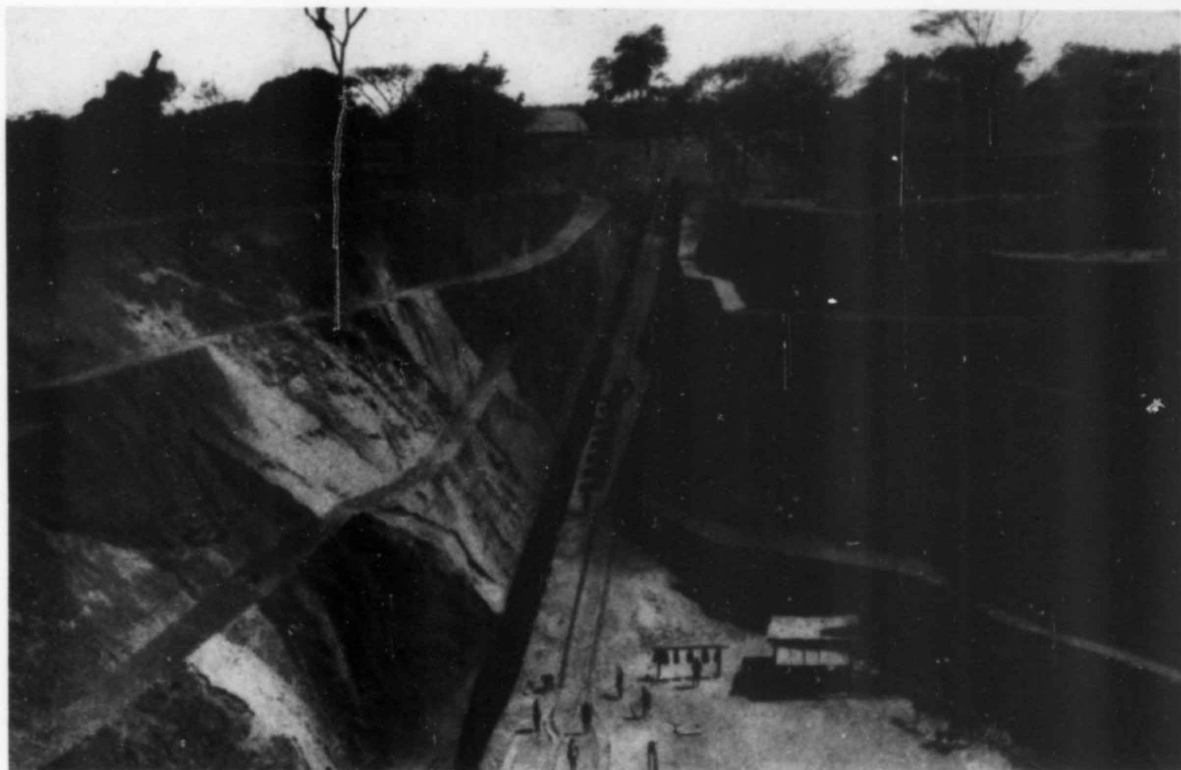
Figure 3. A view of the Shinkolobwe mine, 1930's.
