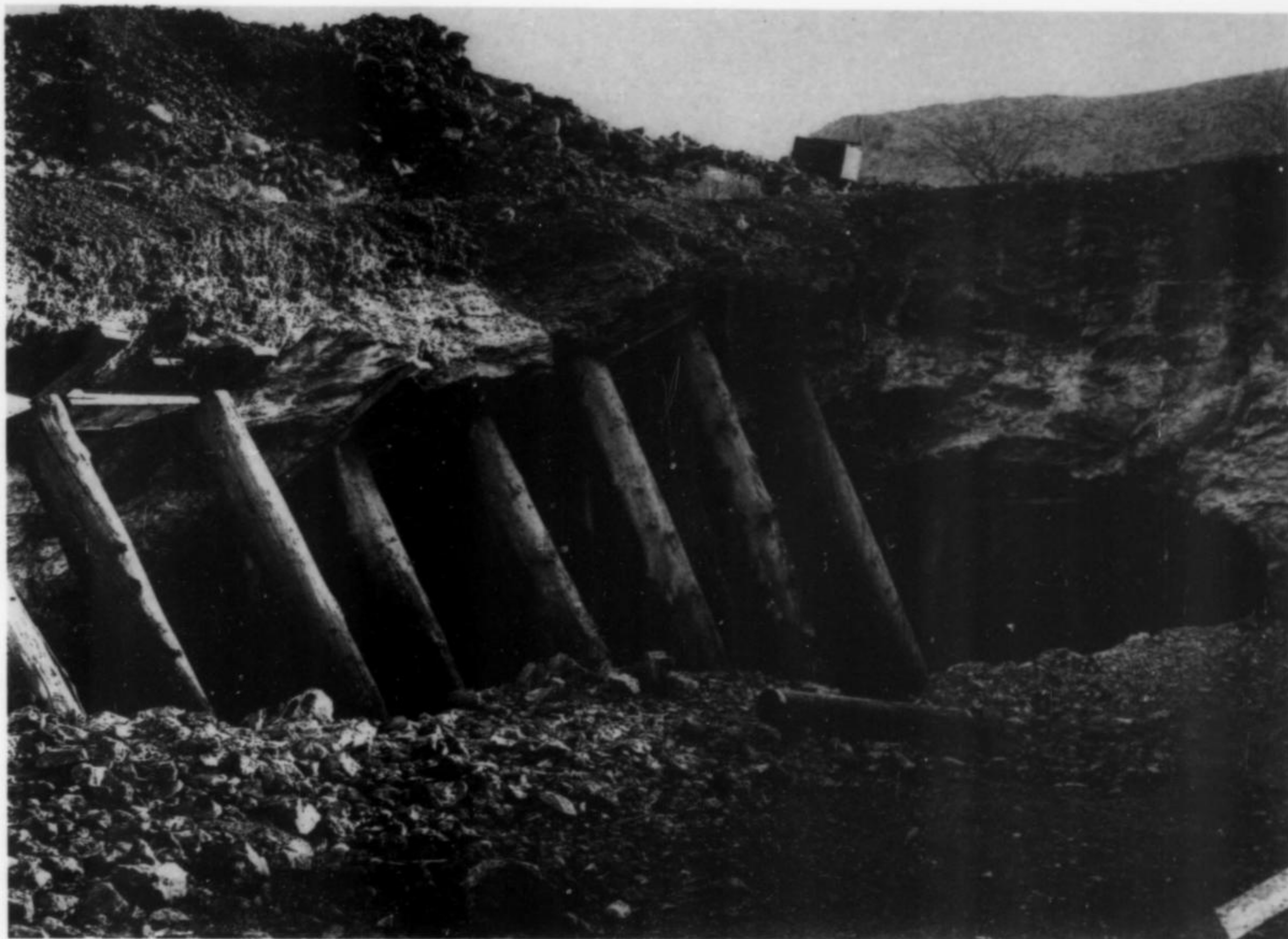
Figure 2. Open cut and stope, Carolina claim, Lake Valley, New Mexico, ca. 1890. This view has often been identified as the Bridal Chamber itself, when in fact it is more likely the location of Daly's exploration drift which eventually broke into the Bridal Chamber several hundred feet away. The ore zone has subsequently been stoped out around the original drift, leaving the opening seen here. Photo Henry Schmidt, NM Bureau of Mines & Mineral Resources Collection, courtesy Richard H. Jahns.
