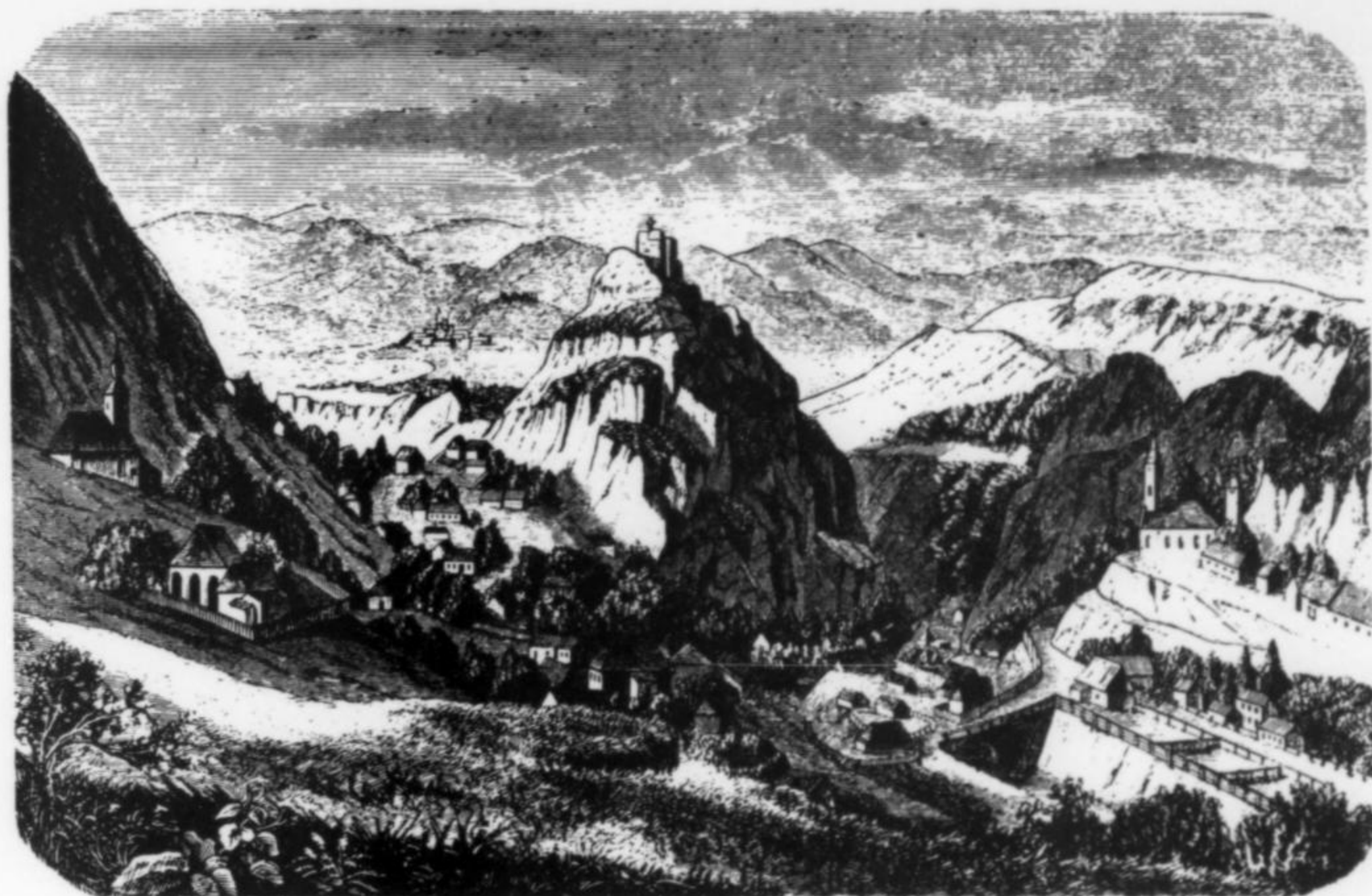
Figure 8. A view of the Nagyag mine area.
