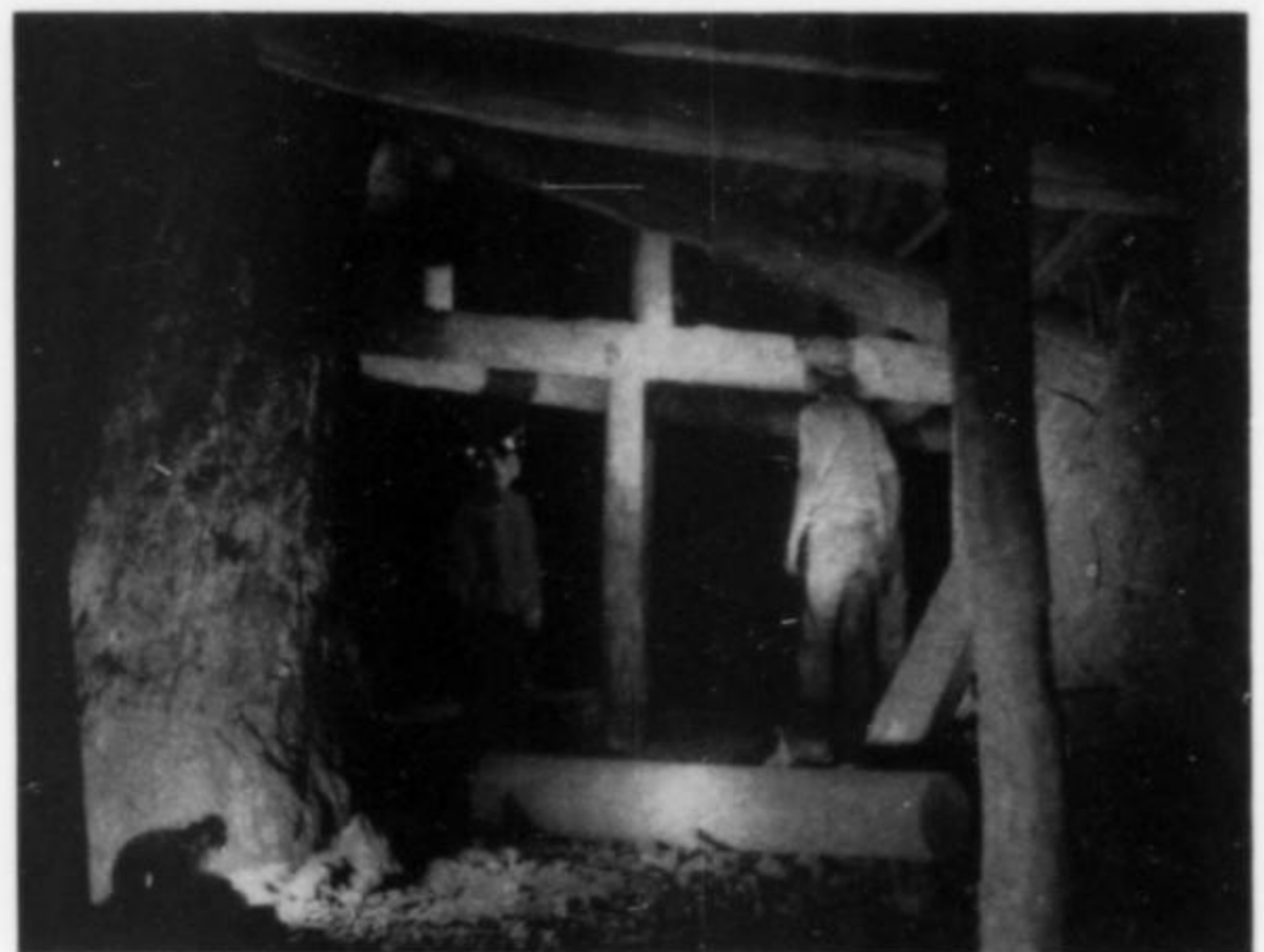
Figure 14. Timbering in the upper workings of the Silver Clip mine, 1979. Photo by G. Bricker.
