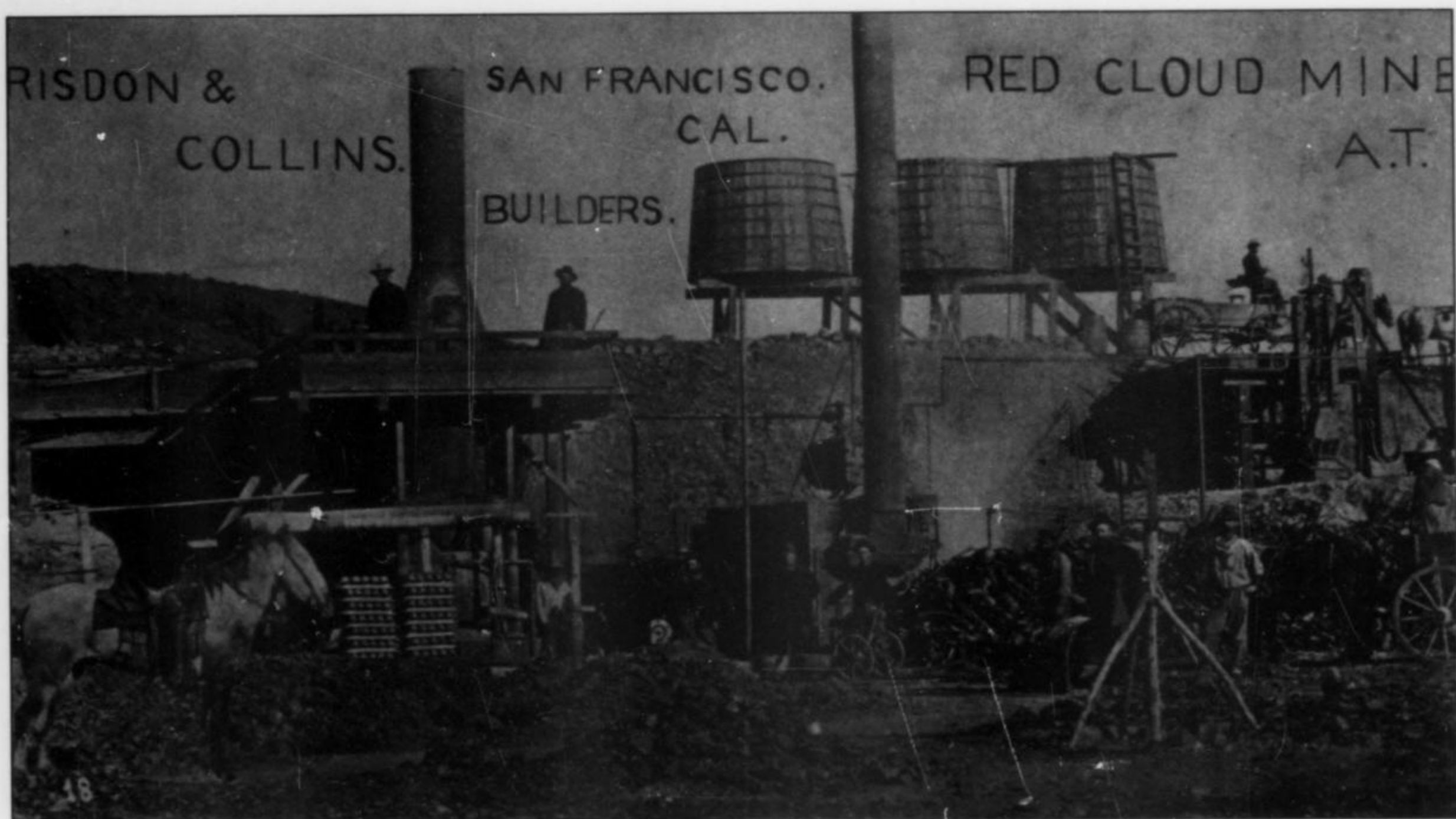
Figure 5. The Black Rock smelter at Norton's Landing, ca. 1881 (not the Red Cloud mine as indicated on the photo). Note man on horseback at left who has been "removed" by an early touch-up artist for reasons that remain a mystery (his leg is still visible). Pigs of silver are stacked just to the right of the horse. Photo courtesy of the California State Library, Sacramento.
