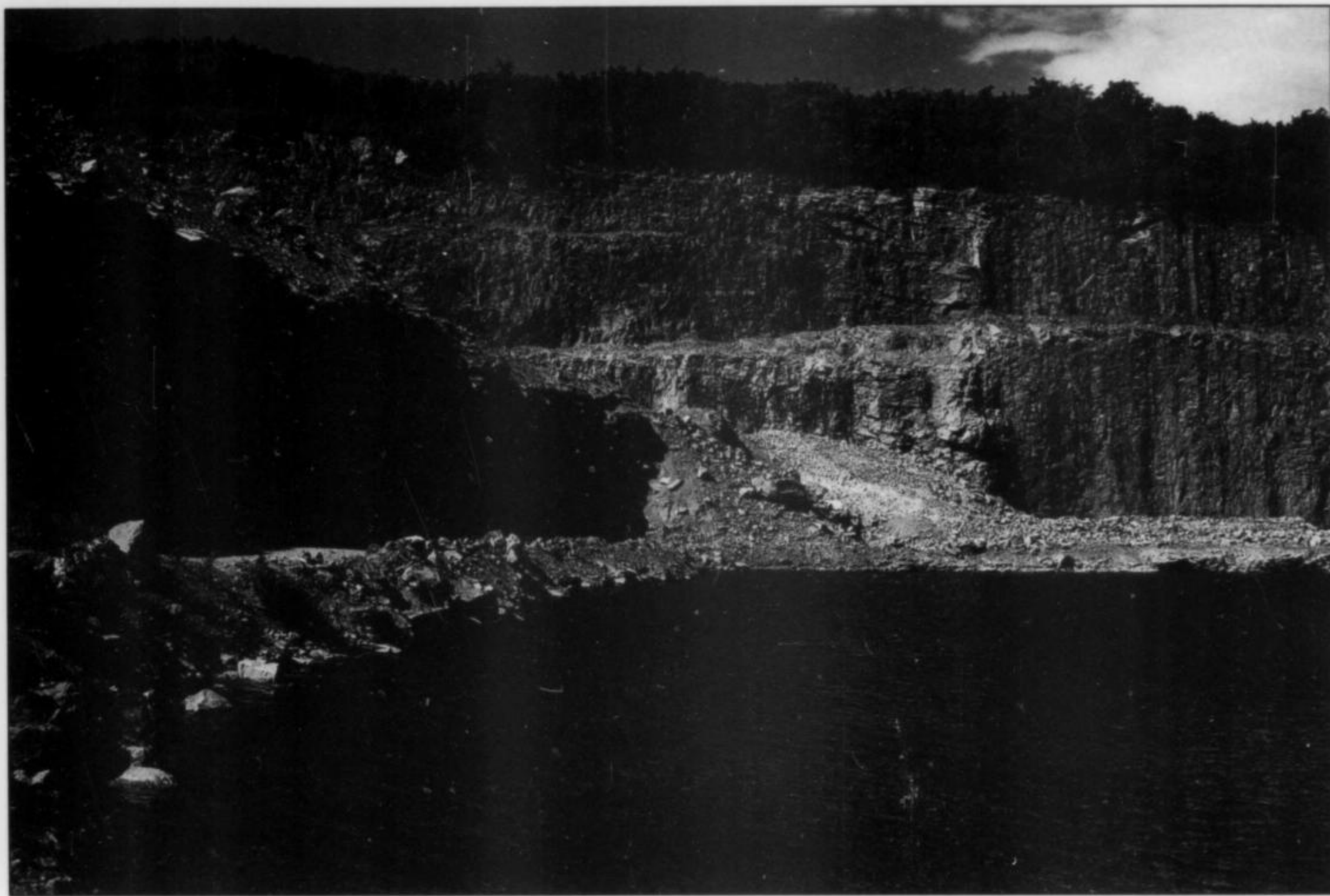
Figure 136. A view of the eastern portion of the Demix quarry showing the wall (left) which separates the Poudrette and Demix quarries. Most of the large siderite pockets were found near this wall. The wall is currently being removed by Poudrette Inc. Photo by L. Horváth.
