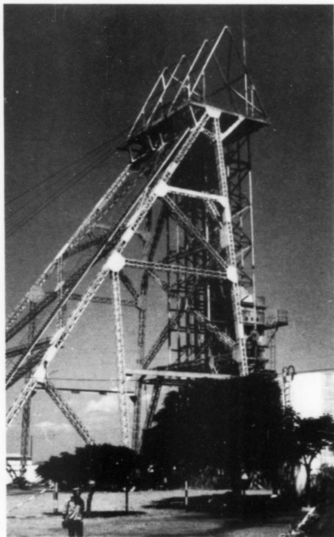
Figure 2. Headgear of the Campbell shaft, Messina mining district. Photo by Terence S. McCarthy.
