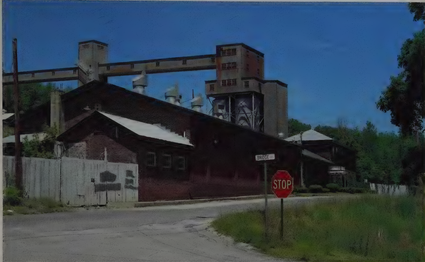
Figure 2. View of Plant Street level from the southeast. The Sterling Hill Exhibit Hall is the large central structure. The ore conveyor and shipping bins are in the background. Photo by Bernard Kozykowski.
