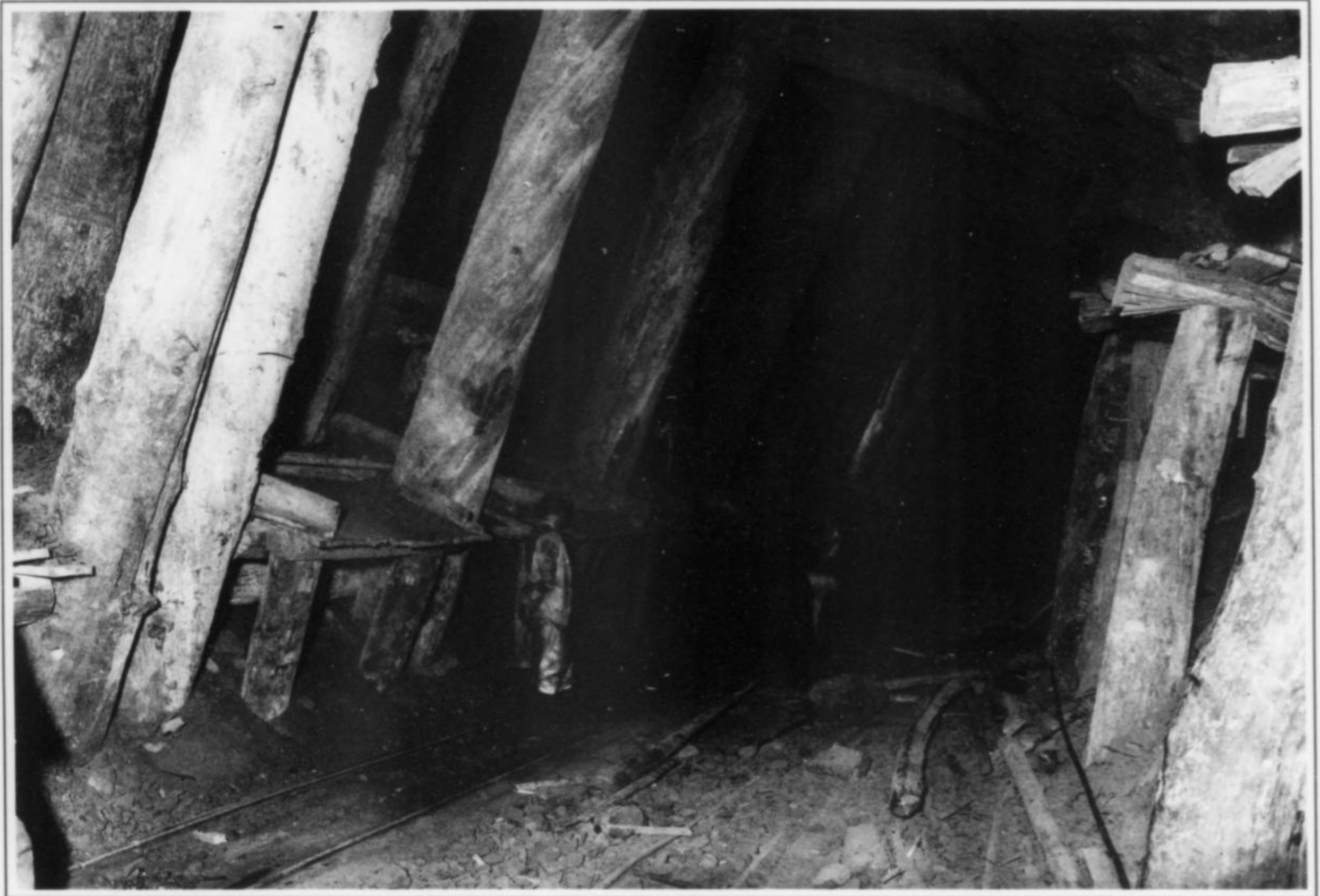
Figure 6. Large timber supports in the Tamarack mine, near the #5 shaft. (MTU Archives)
