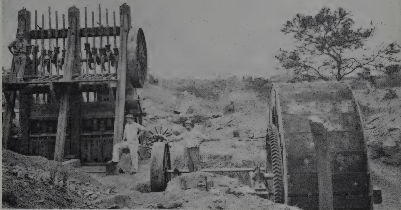
Figure 13. Blue Rock battery. This was a typical 10-stamp mill used to crush the gold-bearing quartz ore. Water channelled in a furrow powered the wheel, which was geared to operate the batteries.
