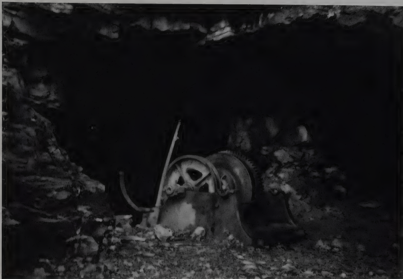
Figure 9. Upper portal of the Monte Cristo mine (photograph by the author).
