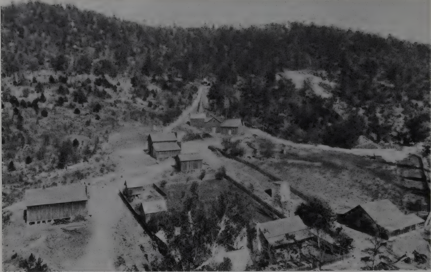
Figure 5. Facilities of the Morning Star mine (Adams, 1904). An elevated railway carried ore to the mill (center). The silver smelter, which was briefly put back into service to produce cement for construction of the mill in 1898, is visible in the lower right.
