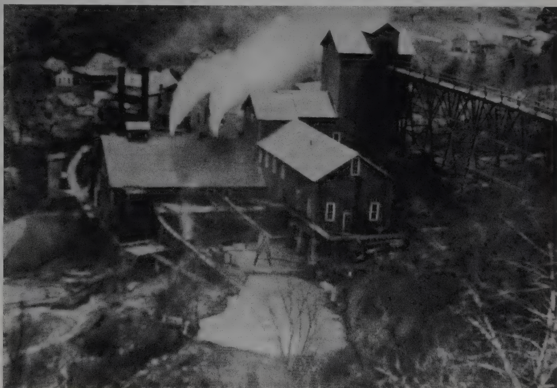
Figure 7. Morning Star concentrator in 1918 after extensive wartime modifications (Engineering and Mining Journal, 16 February 1918).
