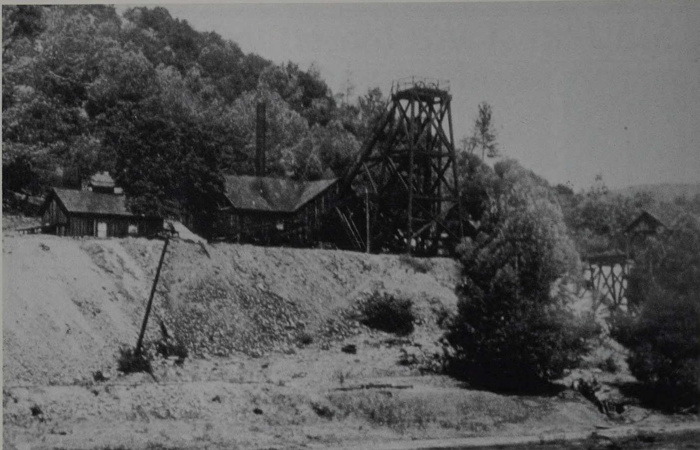
Figure 1. Headframe of the Crystalline mine, 1890's.
