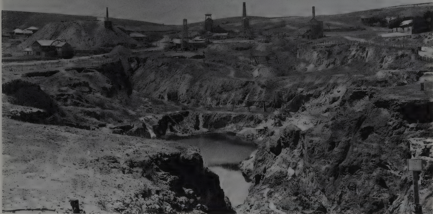
Figure 7. View of the Burra Burra mine and opencut, ca. 1904. Material from the opencut was hauled up in inclined railway to the top of the Mullock dump (left). The tall wooden framework near Morphetts enginehouse is a drilling rig. Peacocks enginehouse, demolished in 1972, is on the extreme right.
