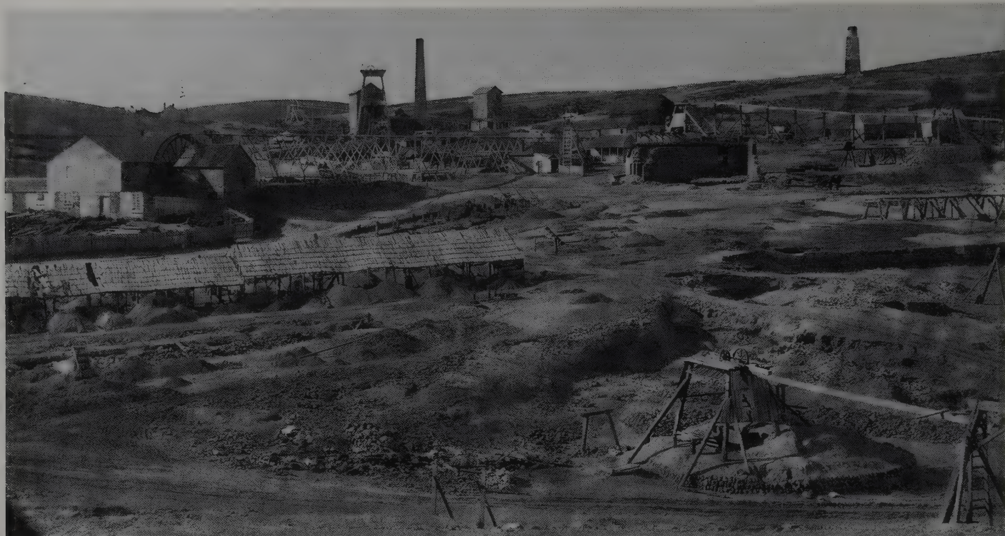
Figure 5. Burra Burra mine, ca. 1868. The view shows Morphetts enginehouse (left) and wind-inghouse. The remains of Schnieders enginehouse can be seen at the right of center. At the left is a crusher house and carpenters' shop powered by a 21-meter waterwheel and an ore dressing shed in the front.
