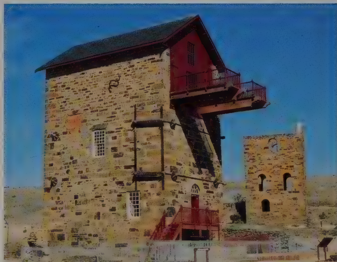
Figure 1. Morphetts enginehouse after its reconstruction in 1986, with Morphetts winding-house in the background.
