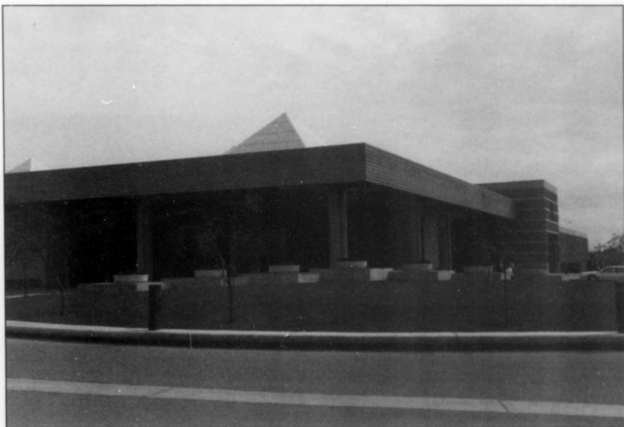
Figure 1. Tucson Convention Center.
