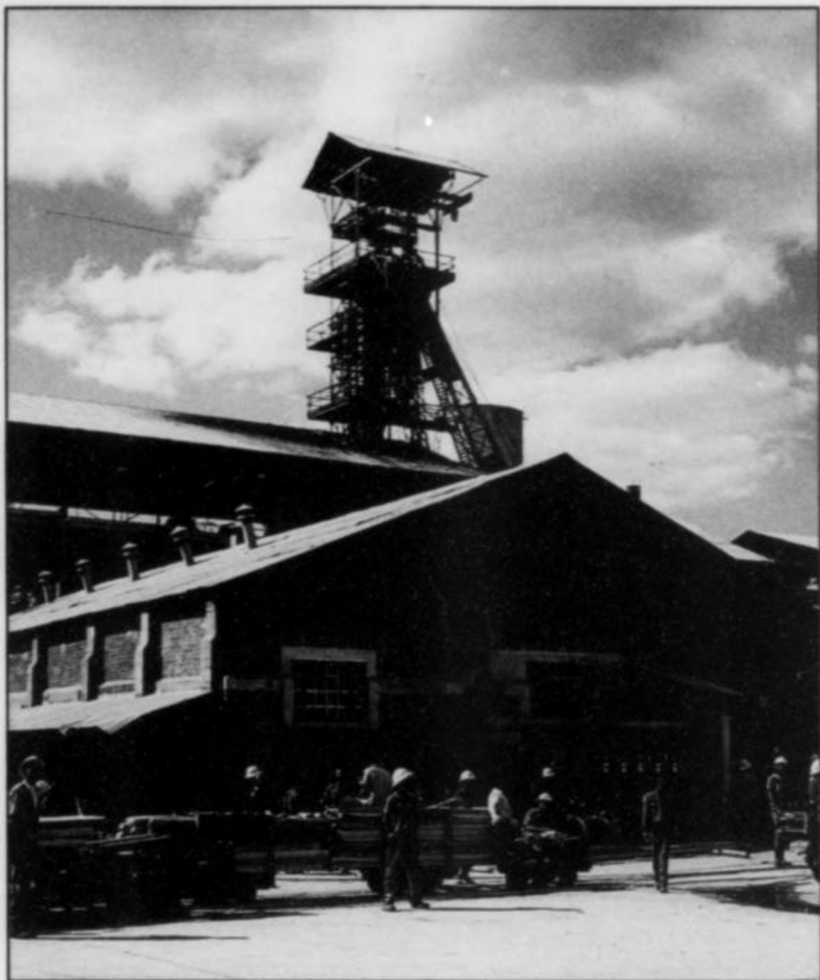
Figure 11. Headframe and mine buildings at Kipushi, shaft II.
