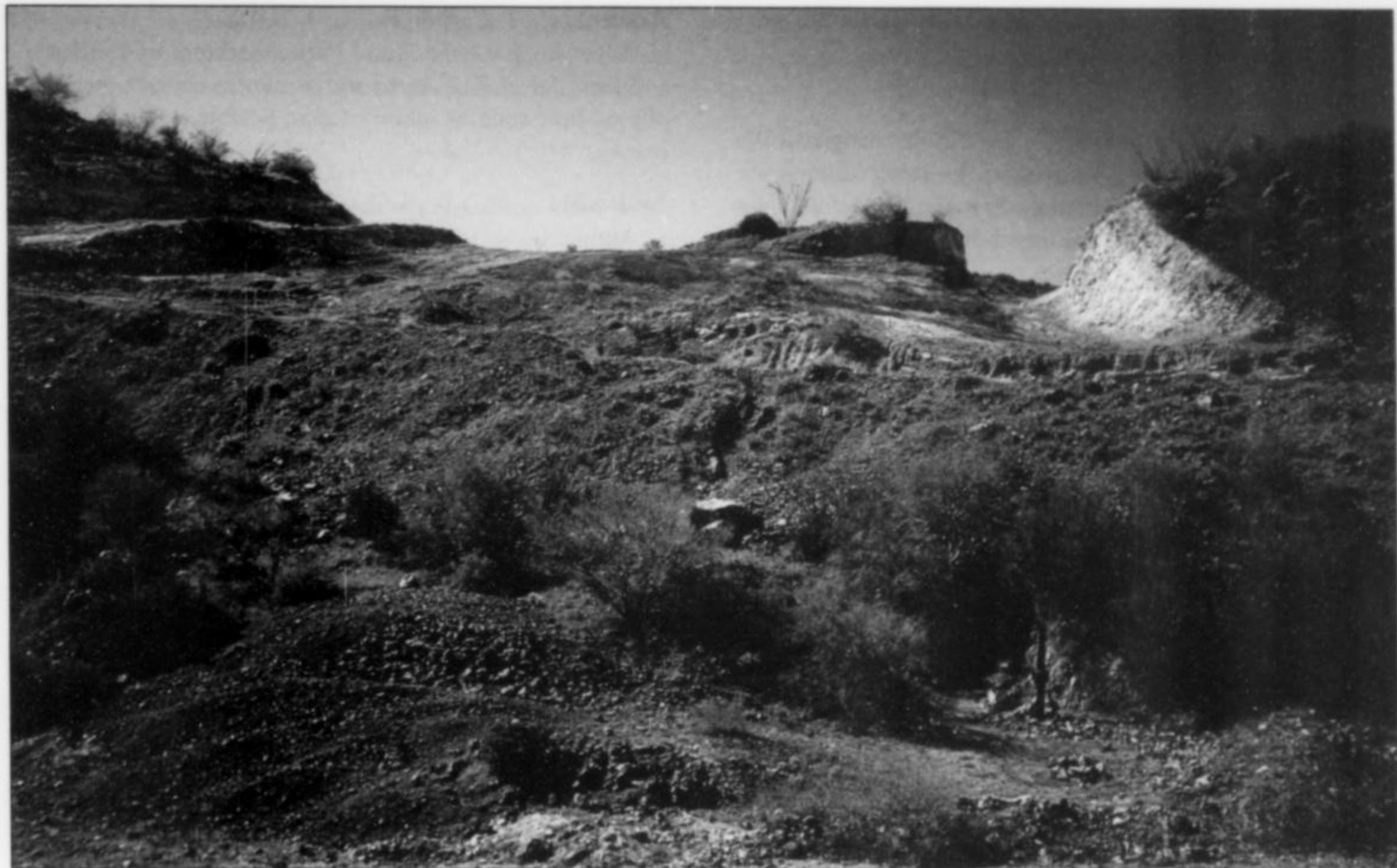
Figure 6. Eastern portal of the Finch mine, and the cut above the mine. K. D. Smith photo.
