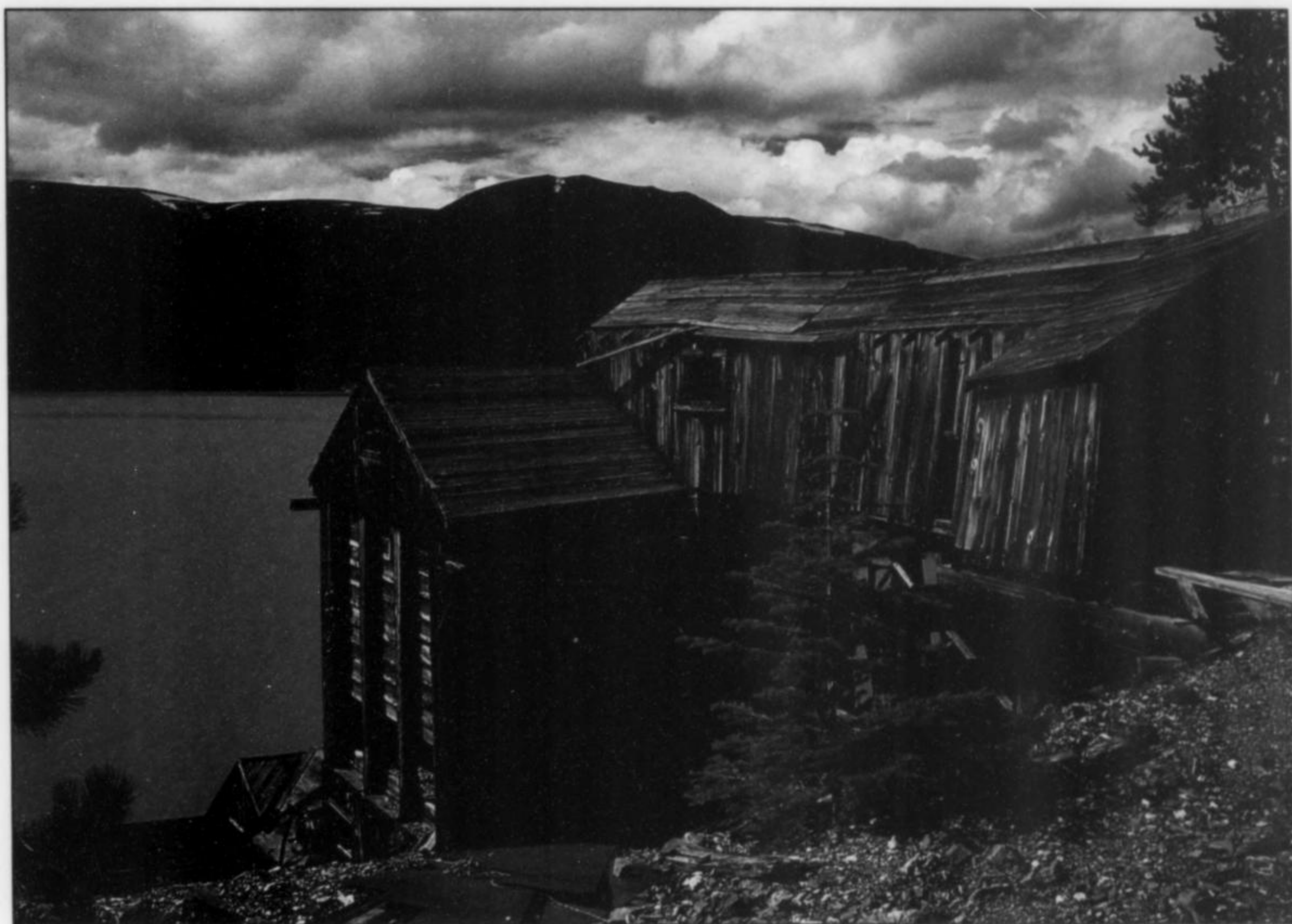
Figure 5. Engineer mine mill on Tagish Lake. Photo by Mark Mauthner.
