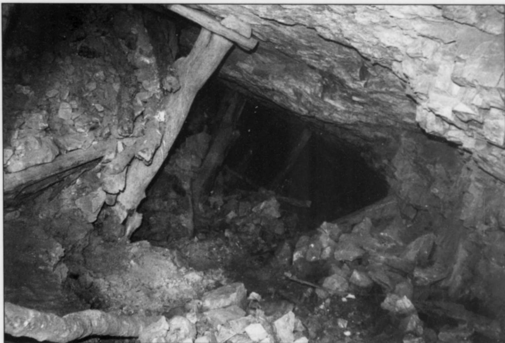
**Figure 8.** Looking down the inclined shaft; note the fallen timbers and back-filled stope on the left. Graham Reeks photo.
