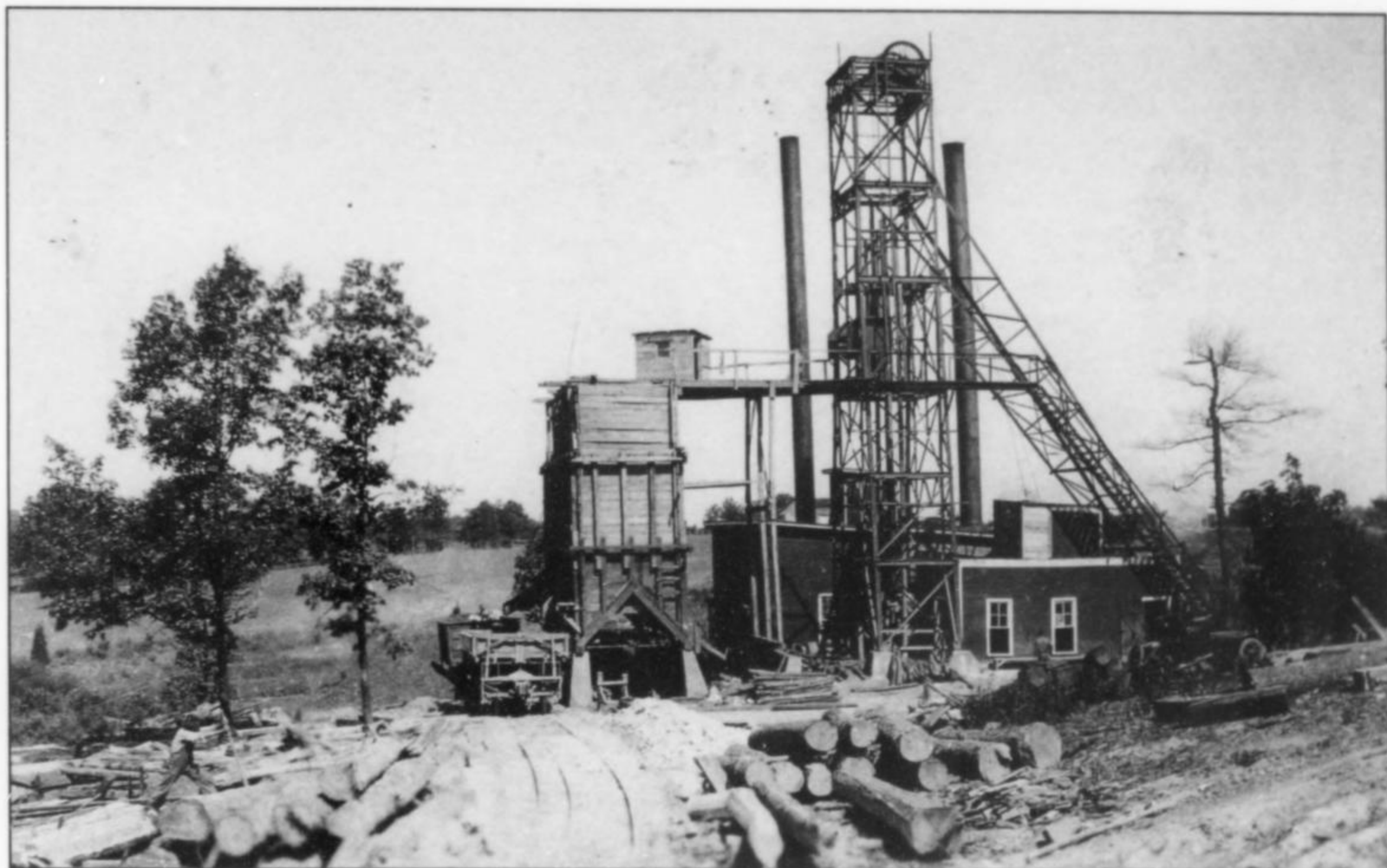
Figure 2. Rosiclare Lead and Fluorspar Company storage bins, ca. 1920. Edwin Reeder photo, courtesy of Mary Hardin.
