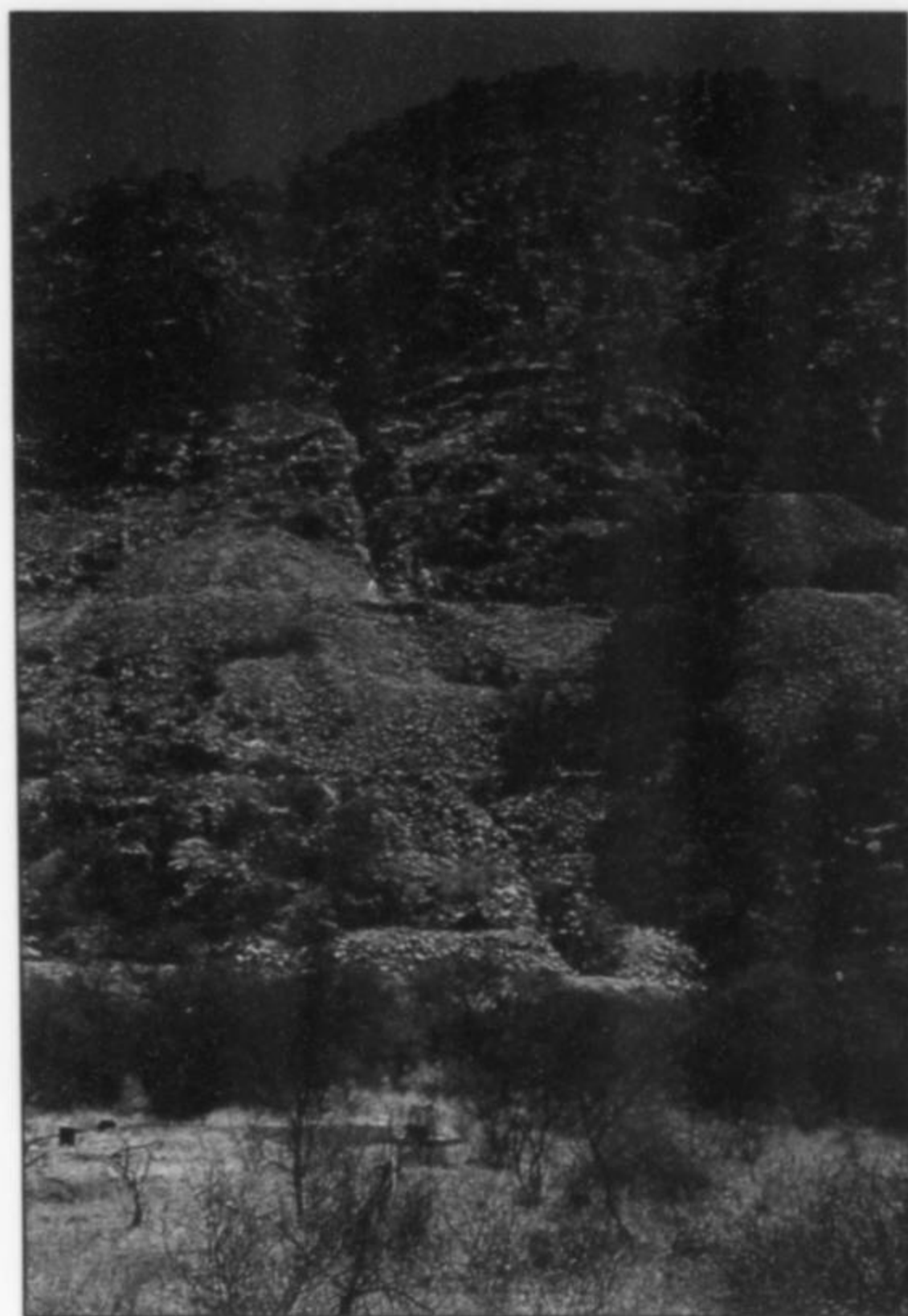
Figure 29. The mined-out mineralization that occurred along a fracture zone at the defunct Baltika mine. Julian Misiewicz photo.
