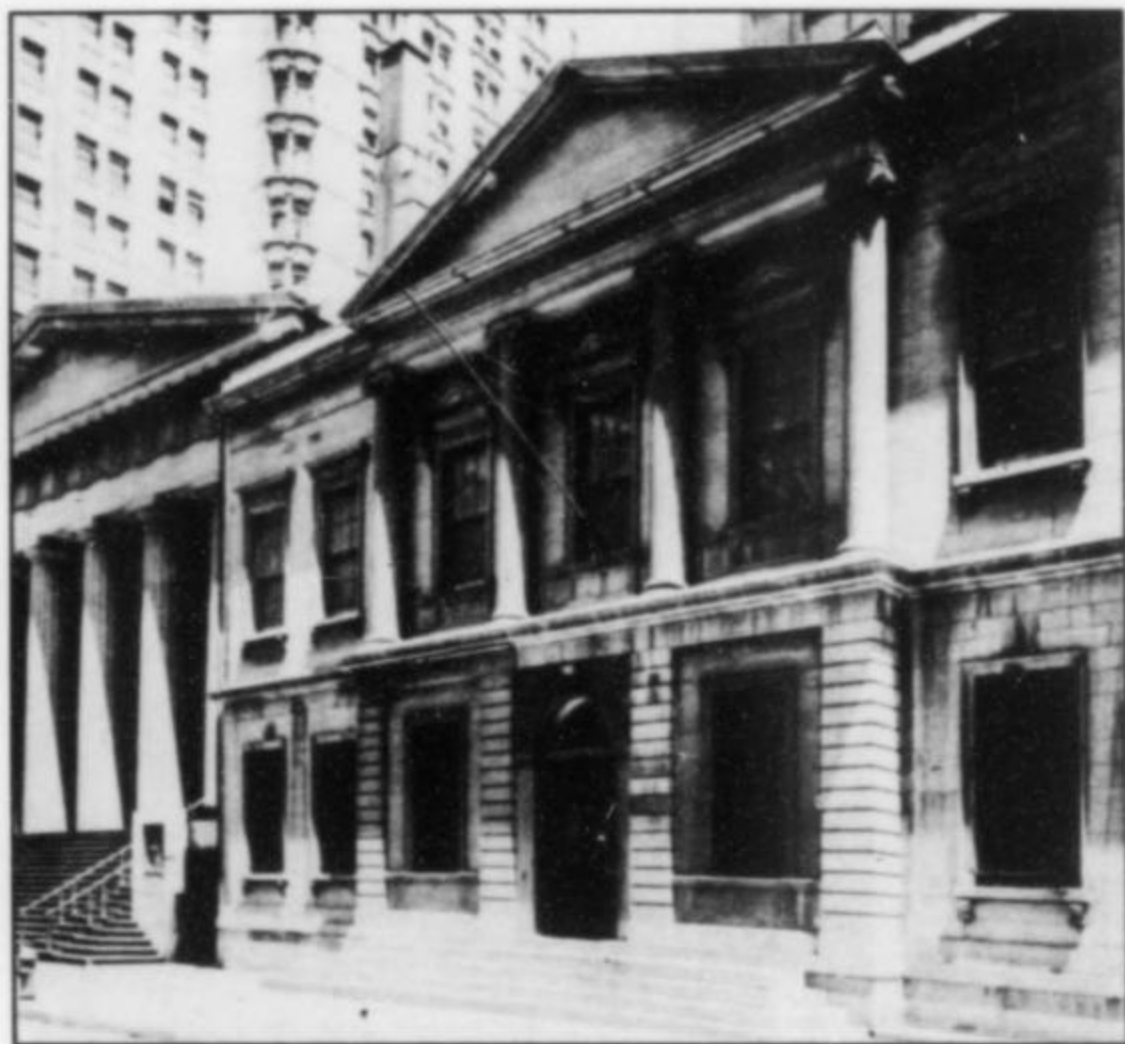
Figure 12. The United States Assay Office (originally the Bank of the United States building), constructed of Inwood B marble from Tuckahoe in 1822. The handsome façade has been preserved and is now on display at the Metropolitan Museum of Art in New York. Immediately to the left is the Custom House, partially built of Inwood A/B marble and still standing at Broad and Wall Streets.
