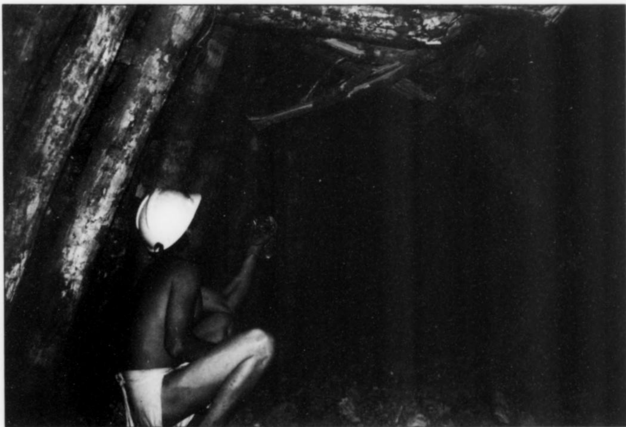
Figure 5. Old workings slowly collapsing in the Amelia mine.
