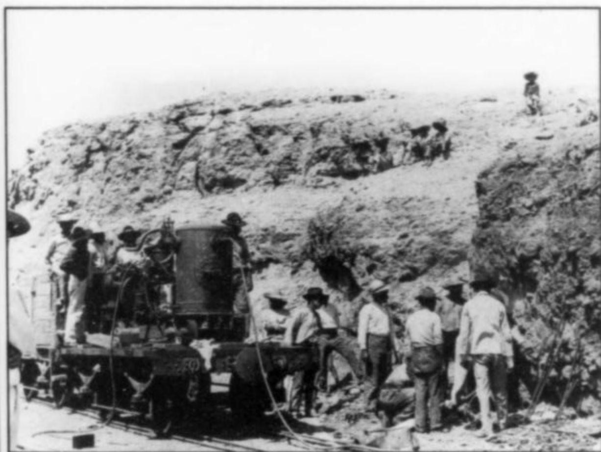
Figure 15. Drilling equipment at Boléo.
