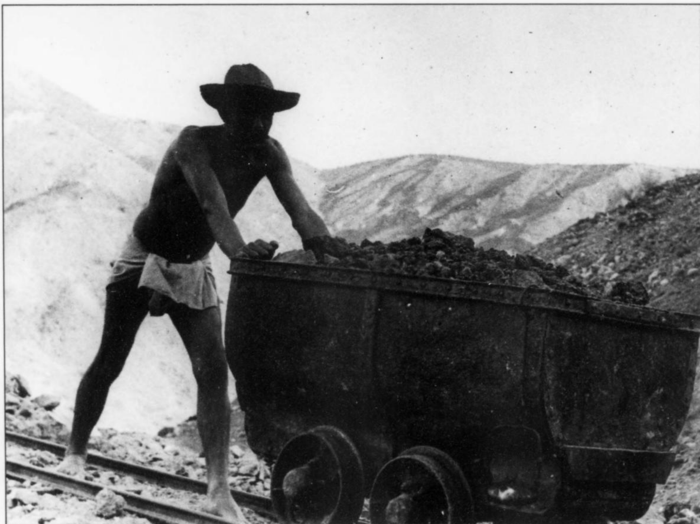
Figure 14. Miner trammung ore at Boléo.
