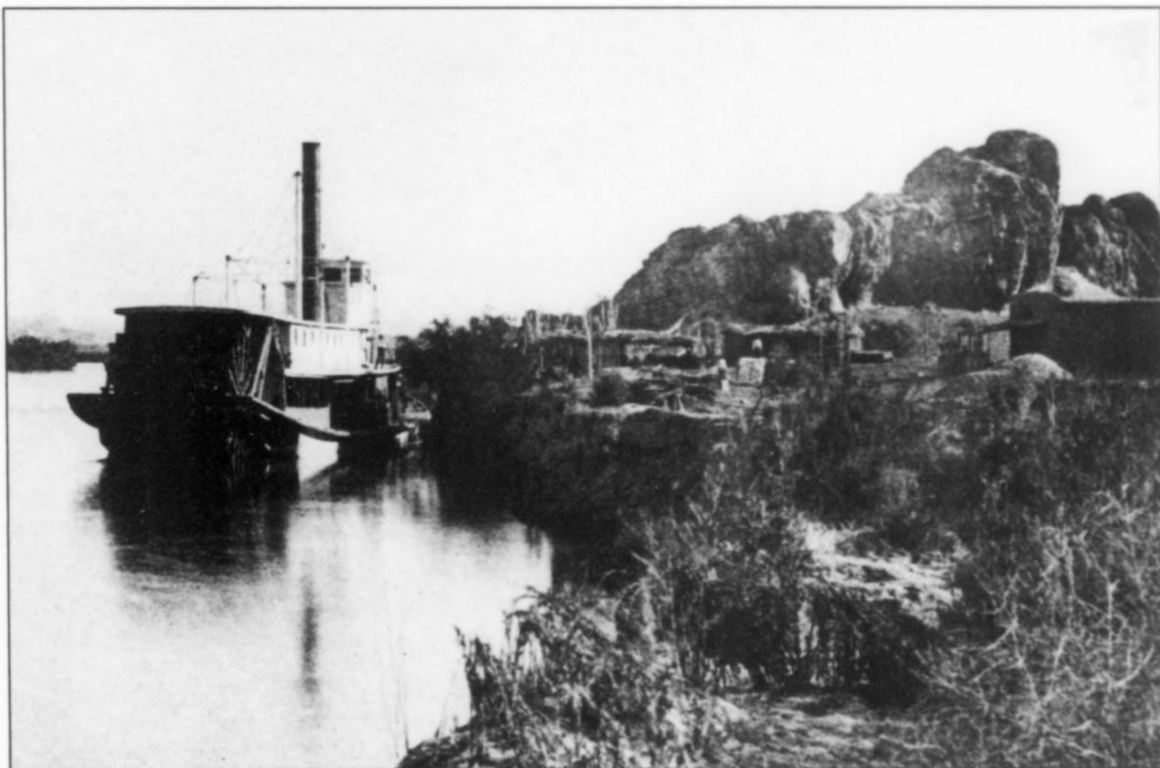
Figure 3. Castle Dome Landing on the Colorado River, 1877. Courtesy Sharlot Hall Museum.
