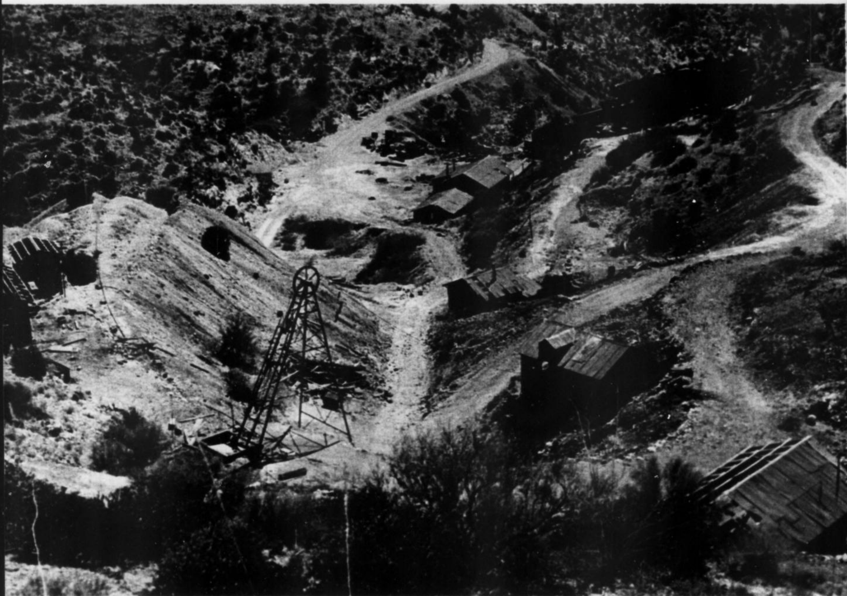
Fig. 3. The 79 mine area as seen from the East. Note cement plug in main shaft in lower left center.
