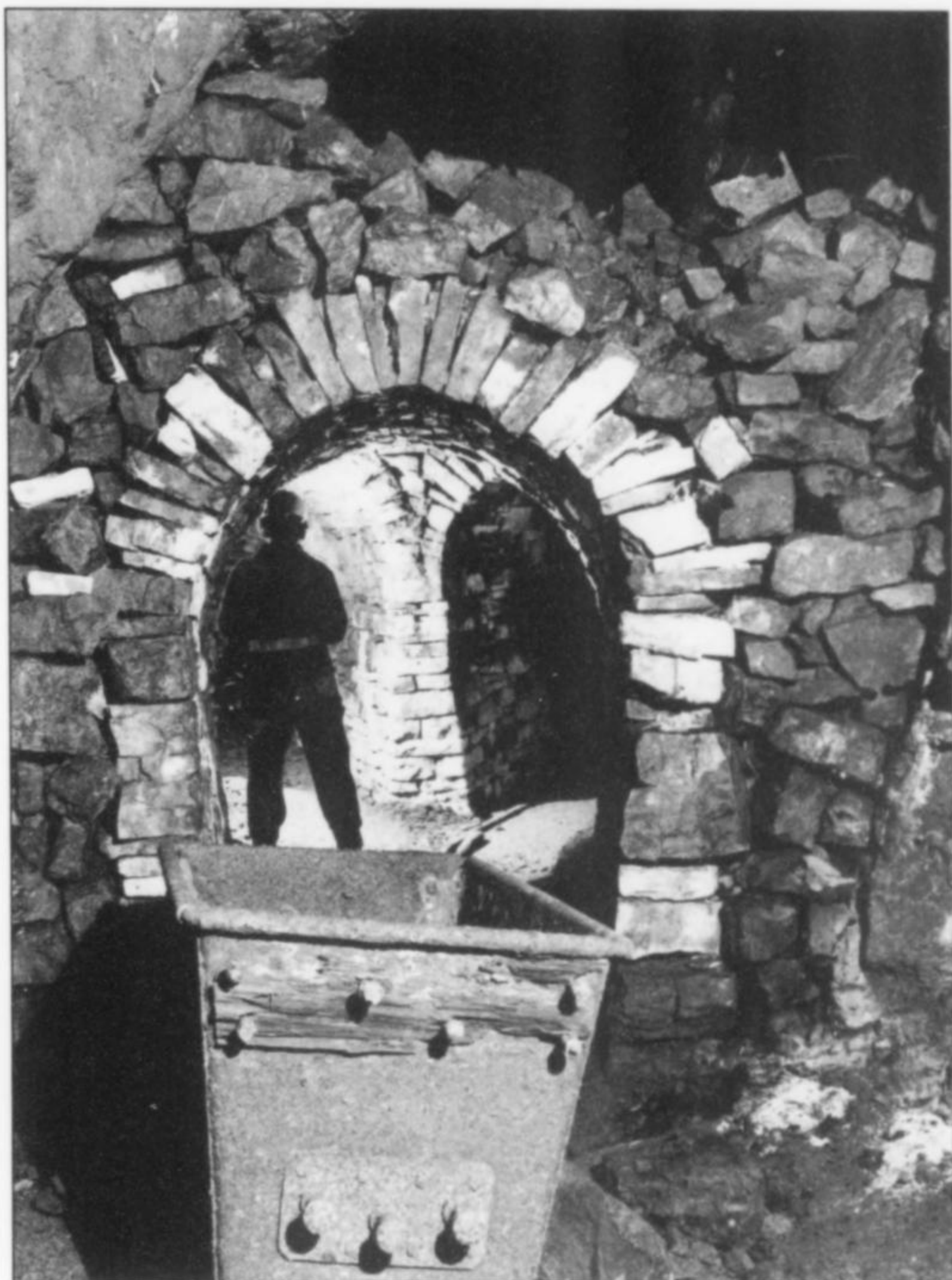
Figure 7. Stone-arched passages in the flat workings. The scarcity of timber meant that most of the passages in the Nenthead mines were stone arched. Waste rock, known locally as "deads," is stacked on top. Photo from the Richard Bird collection.
