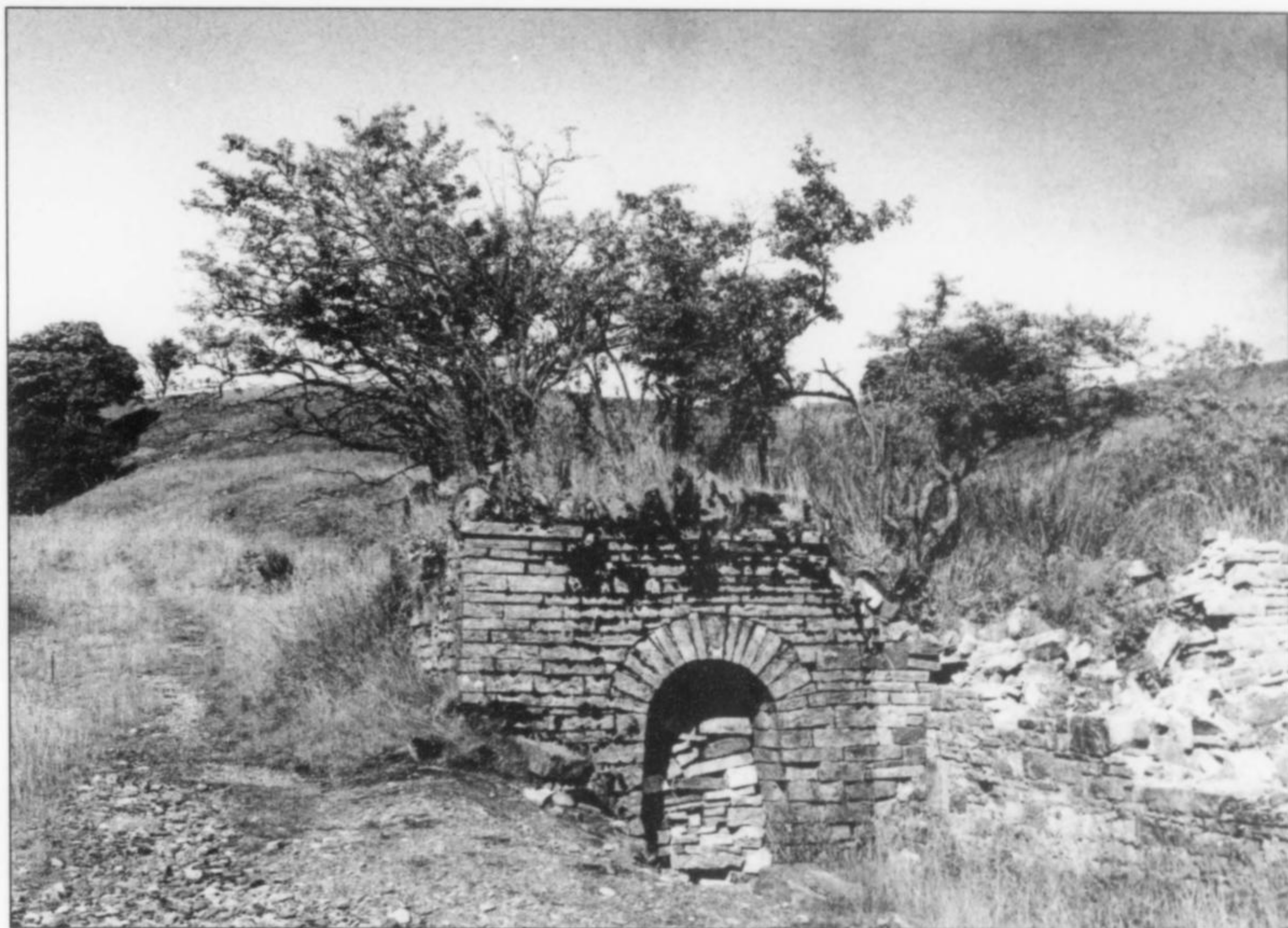
Figure 2. The adit entrance to the Bloomsberry Horse Level, begun sometime prior to 1789 to give access to the ground at the level of the Great Limestone. The photo shows the level as it stood in the late 1970's before the stone walling was removed and replaced by a metal gate. Richard Bird collection.
