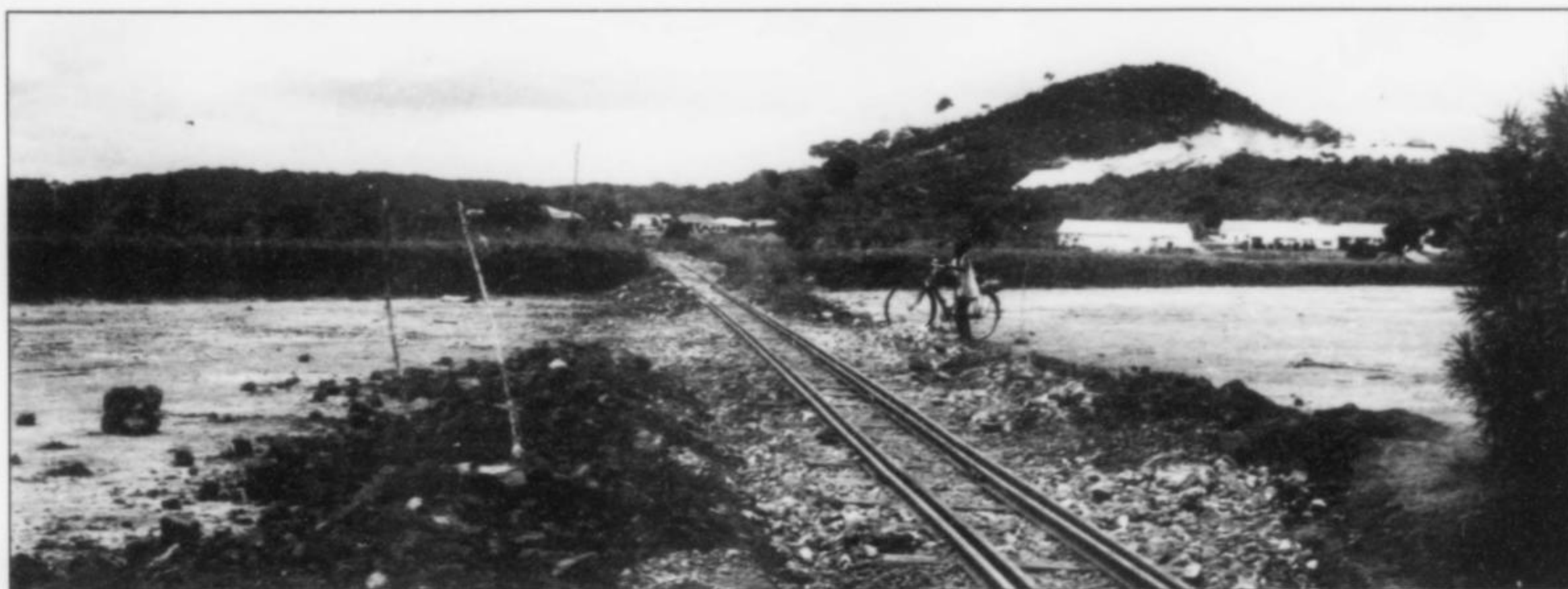
Figure 5. The 7-km narrow-gauge railroad constructed in 1956 by the senior author, connecting the Muiane pegmatite (white gash on the far hillside) with a washing plant on the Metuisse River. Danilo S. Picolo photo.
