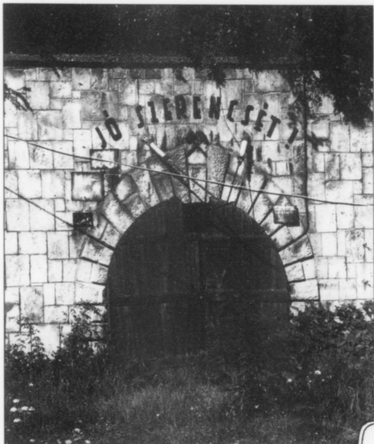
Figure 20. Portal of the haulage tunnel in 1994. R. Triebel photo.
