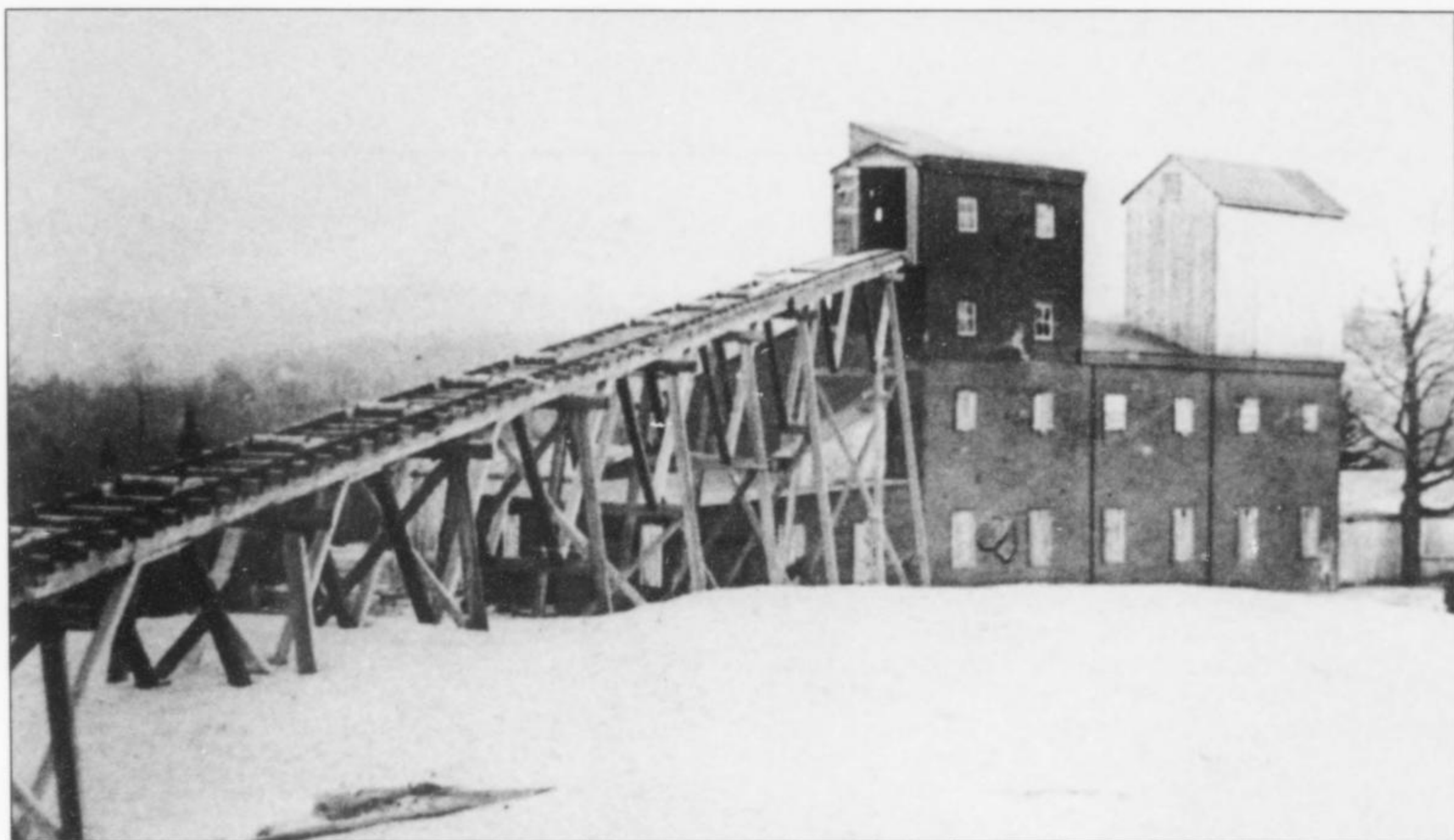
Figure 8. Forty-foot-high hoisting house and stamp mill at the Williams shaft, Bristol. Photo courtesy of John Pawloski.
