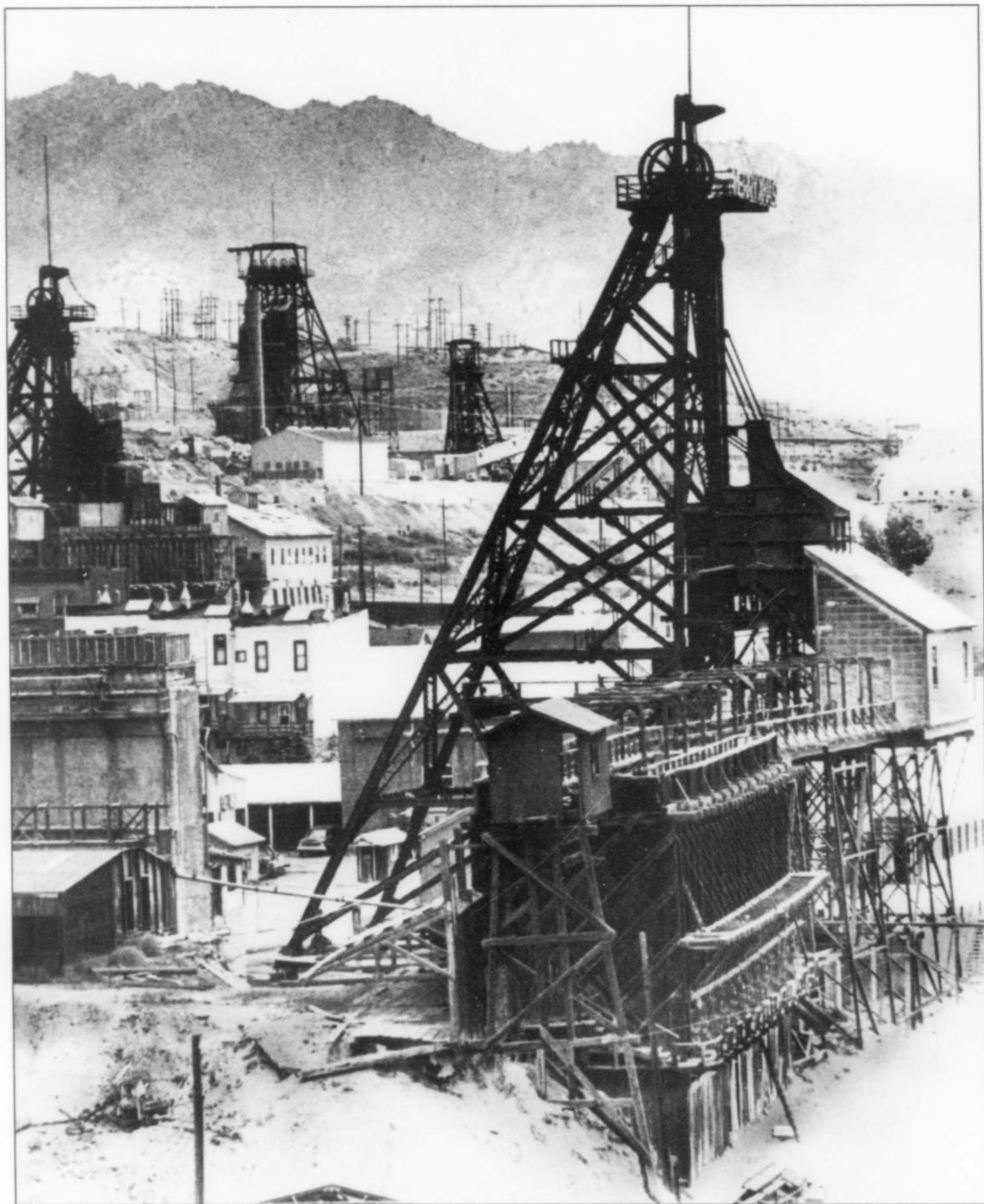
Figure 1. Steel headframes of the Original (foreground), Kelley #1 (center-background), Steward (left-background) and Kelley #2 (right-background) mines, Butte, ca. 1965. World Museum of Mining photo.
