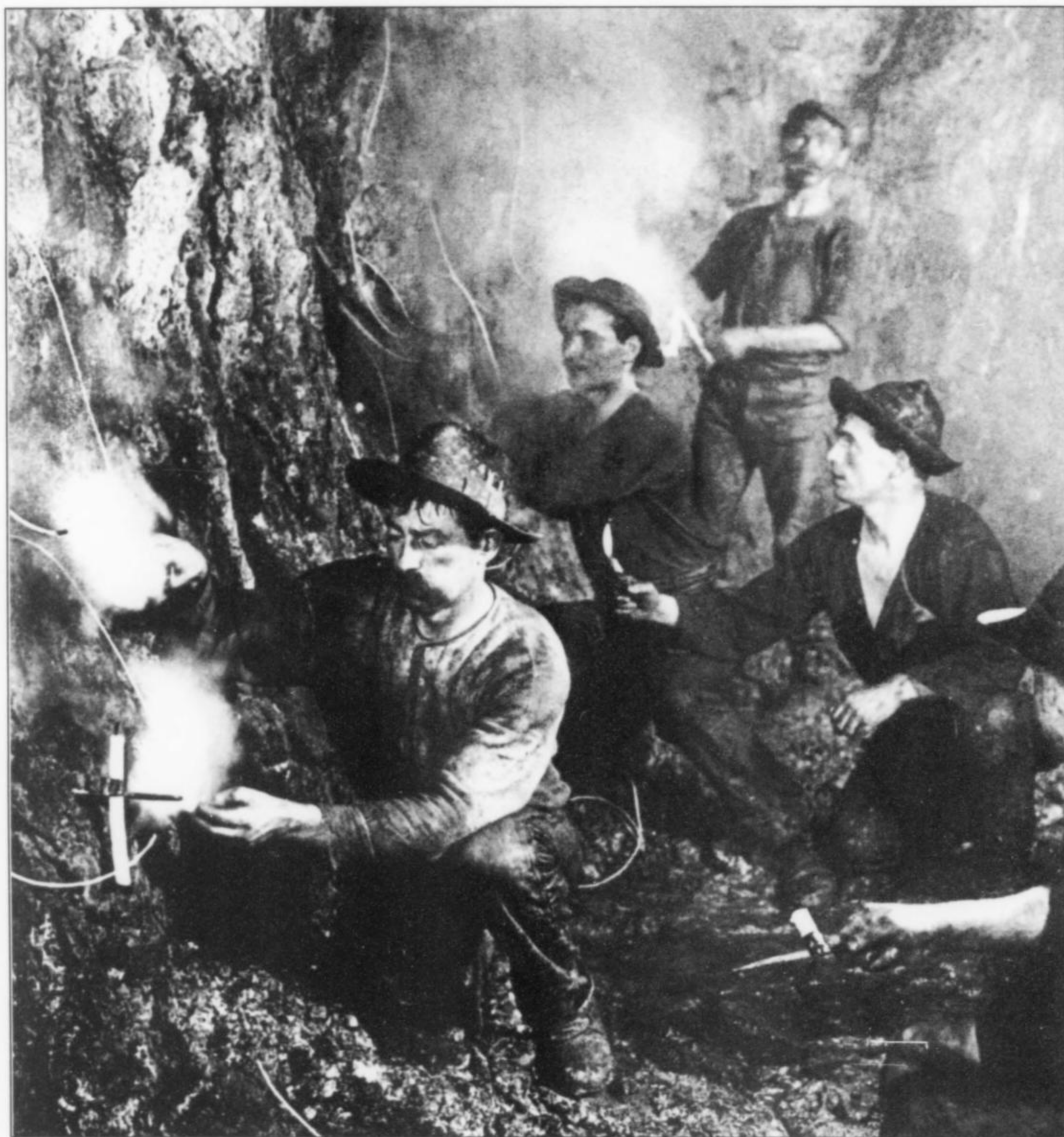
Figure 2. Miners lighting fuses 900 feet under the Butte Post Office, in the Steward mine, 1897. World Museum of Mining photo.
