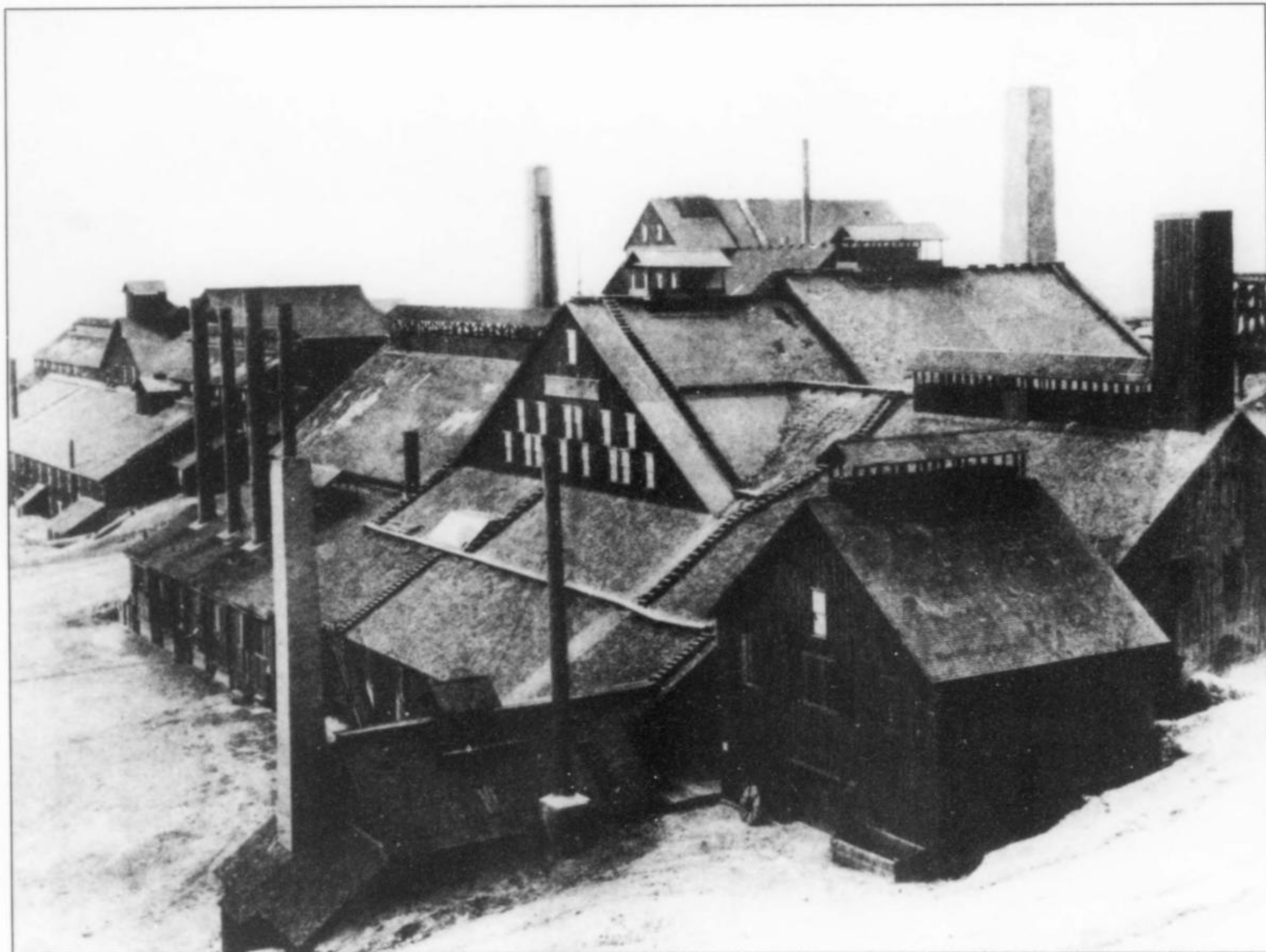
Figure 20. Surface buildings of the Alice mine, 1880. World Museum of Mining photo.
