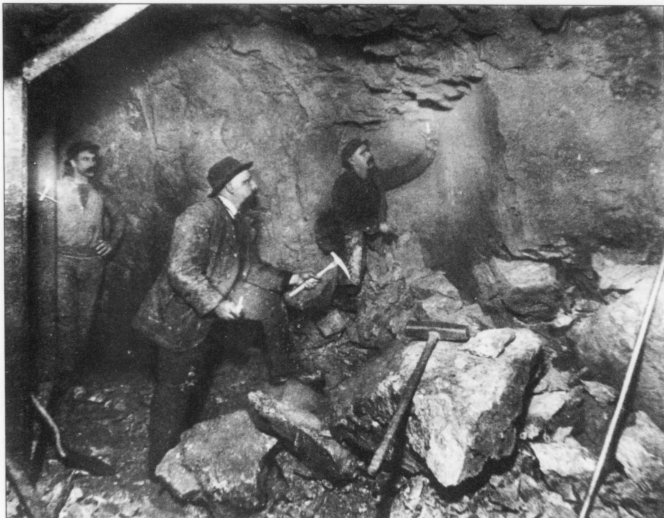
Figure 7. Inspecting the working face after a blast, Leonard mine ca. 1879. World Museum of Mining photo.
