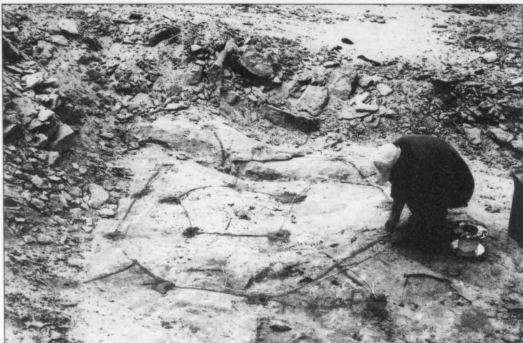
Figure 13. (right) Preparing an area at the Mile 72 site for blasting, 1999. Chris Johnston photo.
