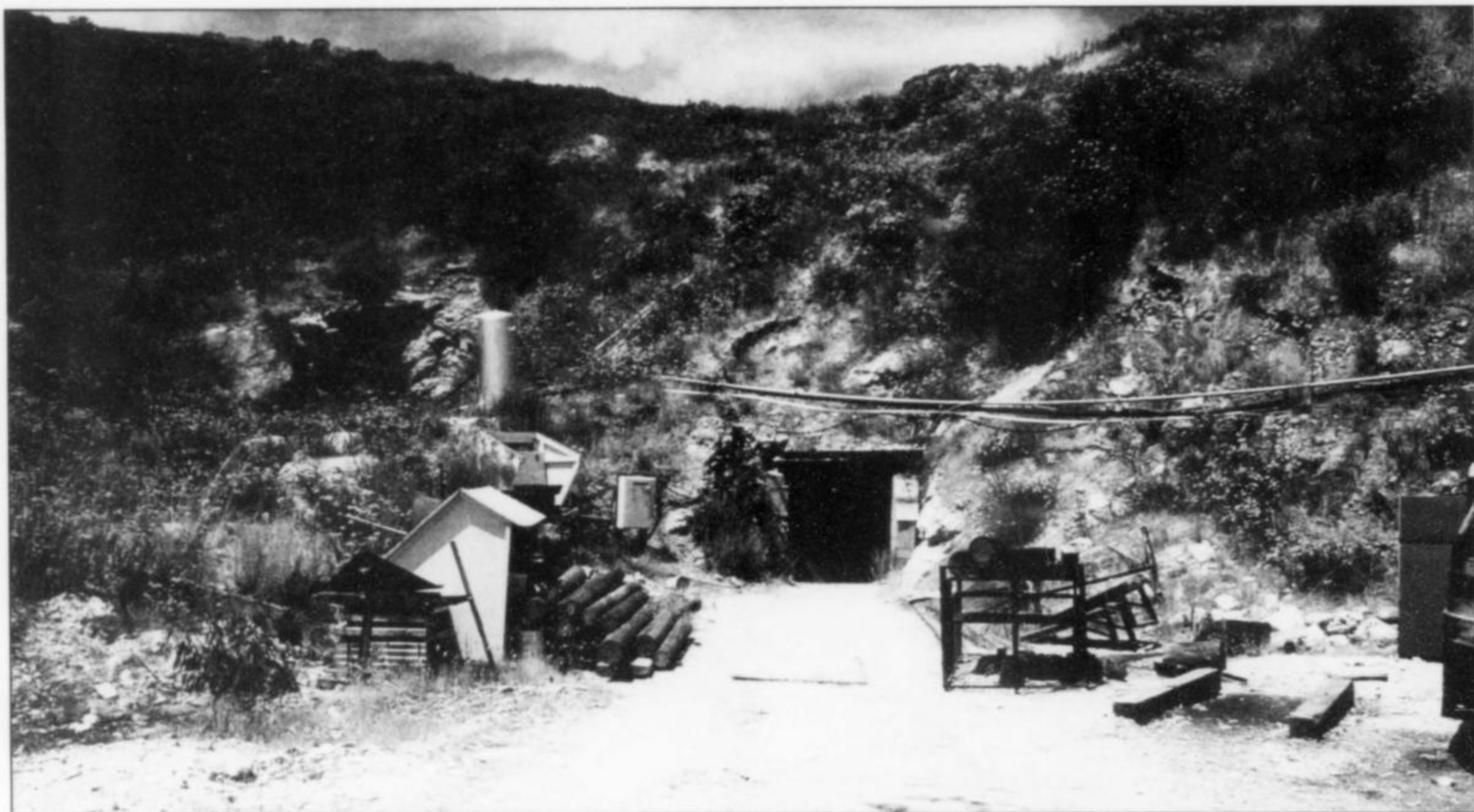
Figure 24. The main portal of the Stewart mine, 1997. Jesse Fisher photo.
