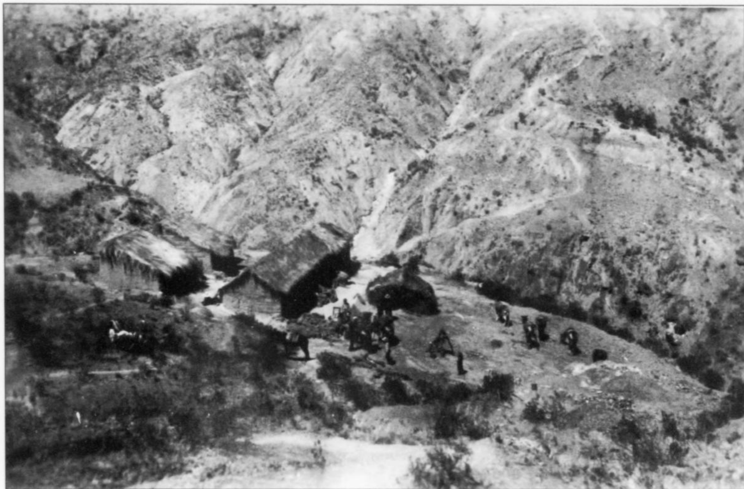
Figure 2. Ore sacks being loaded onto mules at the Surumi Pampa camp at Pacajake in 1935. (Photo courtesy of Hans Block Jr.)
