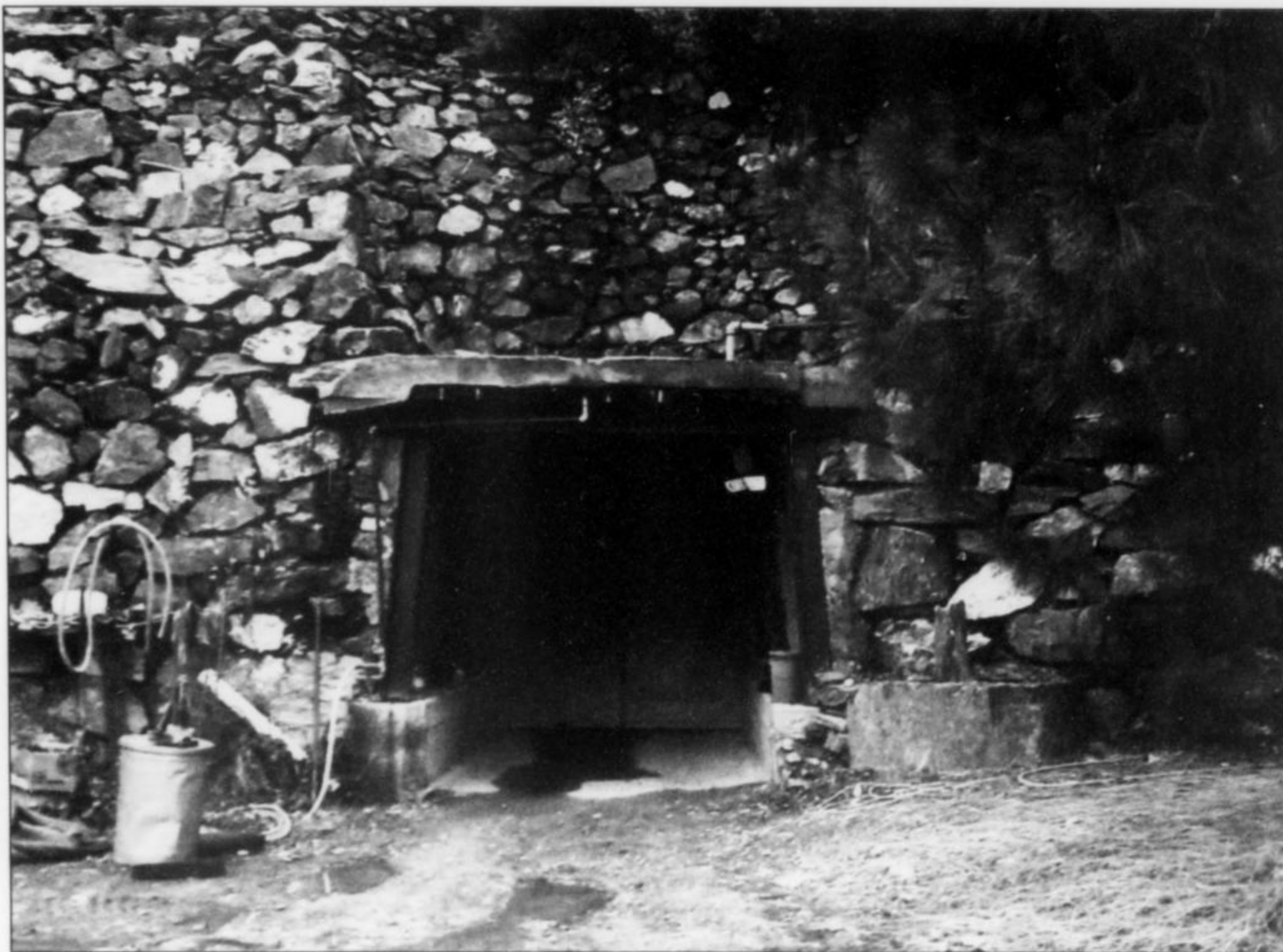
Figure 3. Adit entrance to the Eagle's Nest mine. Robert Cook photo.
