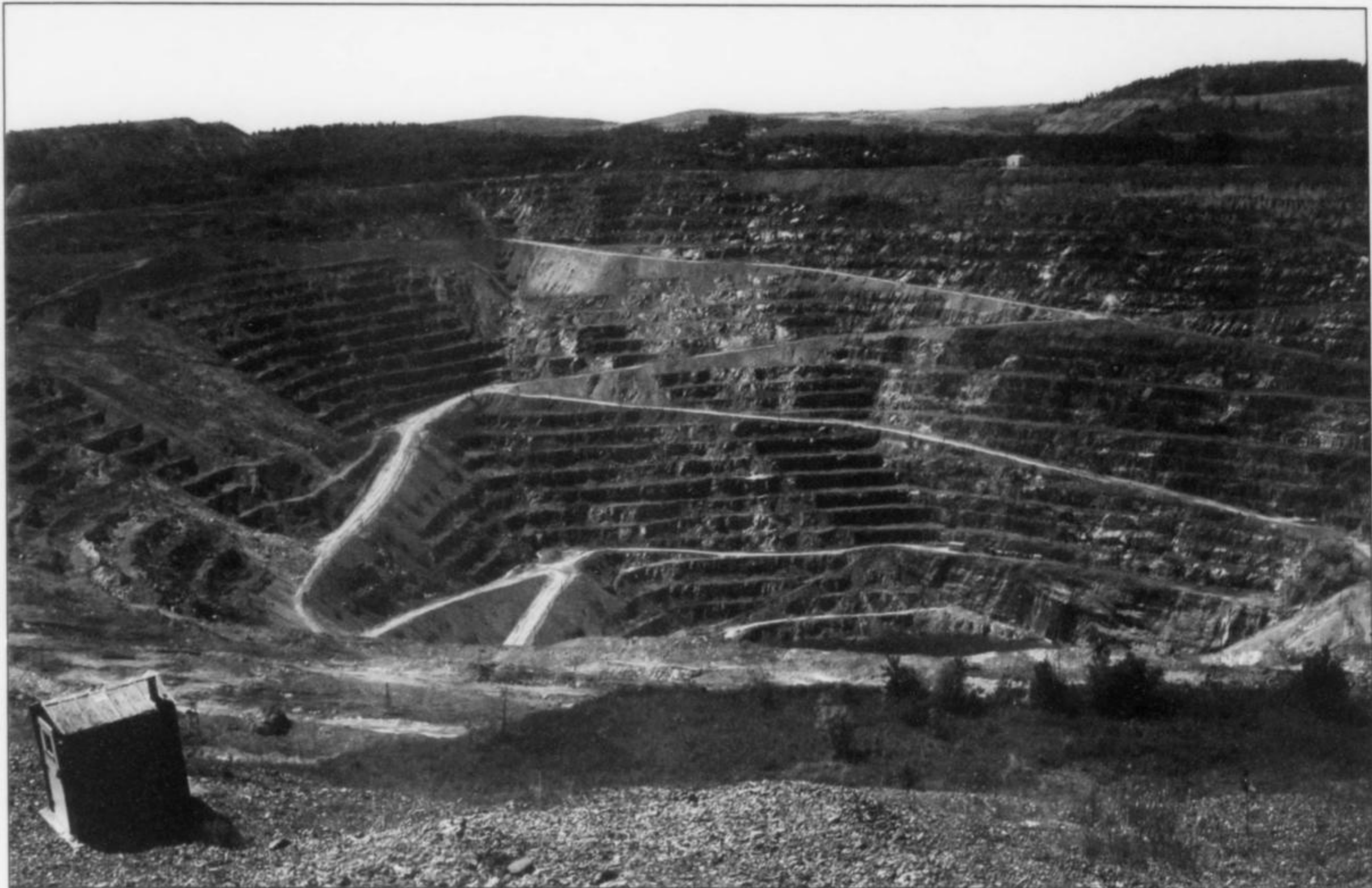
Figure 2. The Jeffrey mine in June 2003. The bottom of the pit is already flooded to a depth of about 300 feet. Amabili photo.
