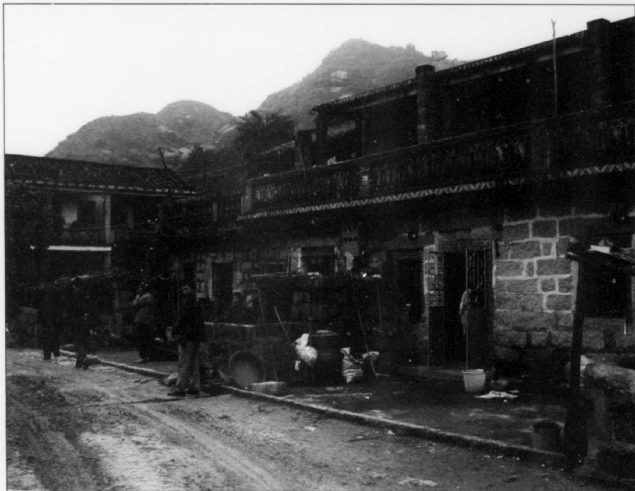
Figure 3. All of the houses in Tongbei are constructed of granite, the principal product of the area. Ottens photo.
