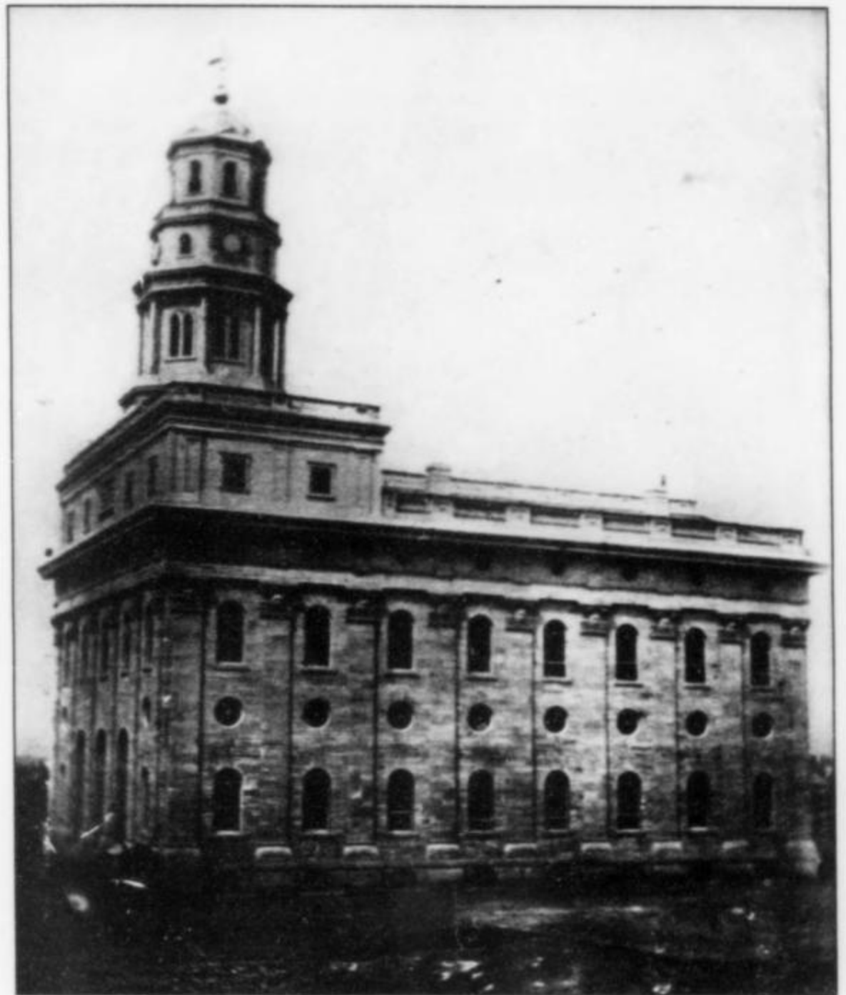
Figure 4. The Mormon Temple at Nauvoo, Illinois, constructed of Mississippiian Keokuk Limestone; 1846 photo courtesy of the Church of Jesus Christ of Latter-Day Saints.
