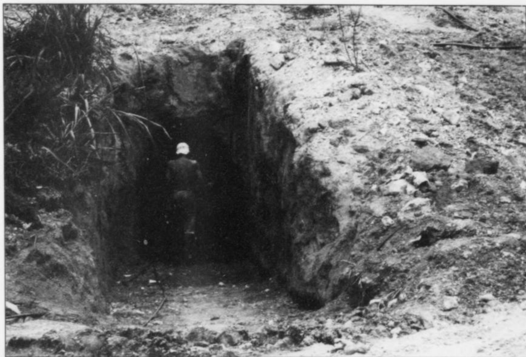
Figure 3. In a tunnel entrance to the Santa Rosa mine, Itambacuri, Minas Gerais.
