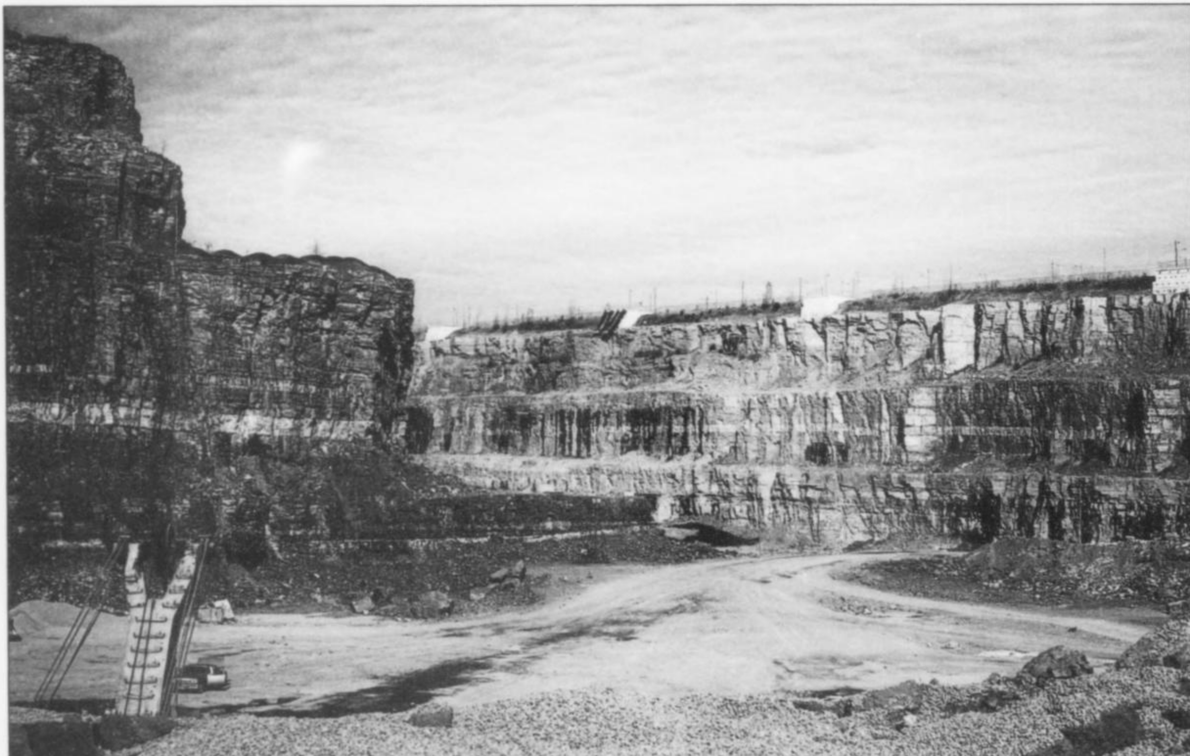
Figure 3. A view of the Francon quarry looking north from the "alcove" area. L. Horváth photo, 1982.
