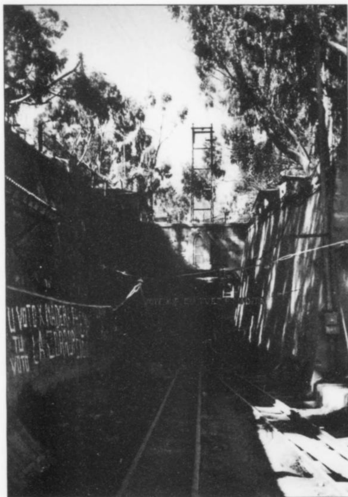
Figure 6. The portal of the Siglo XX Tunnel today. Hyrsi photo.
