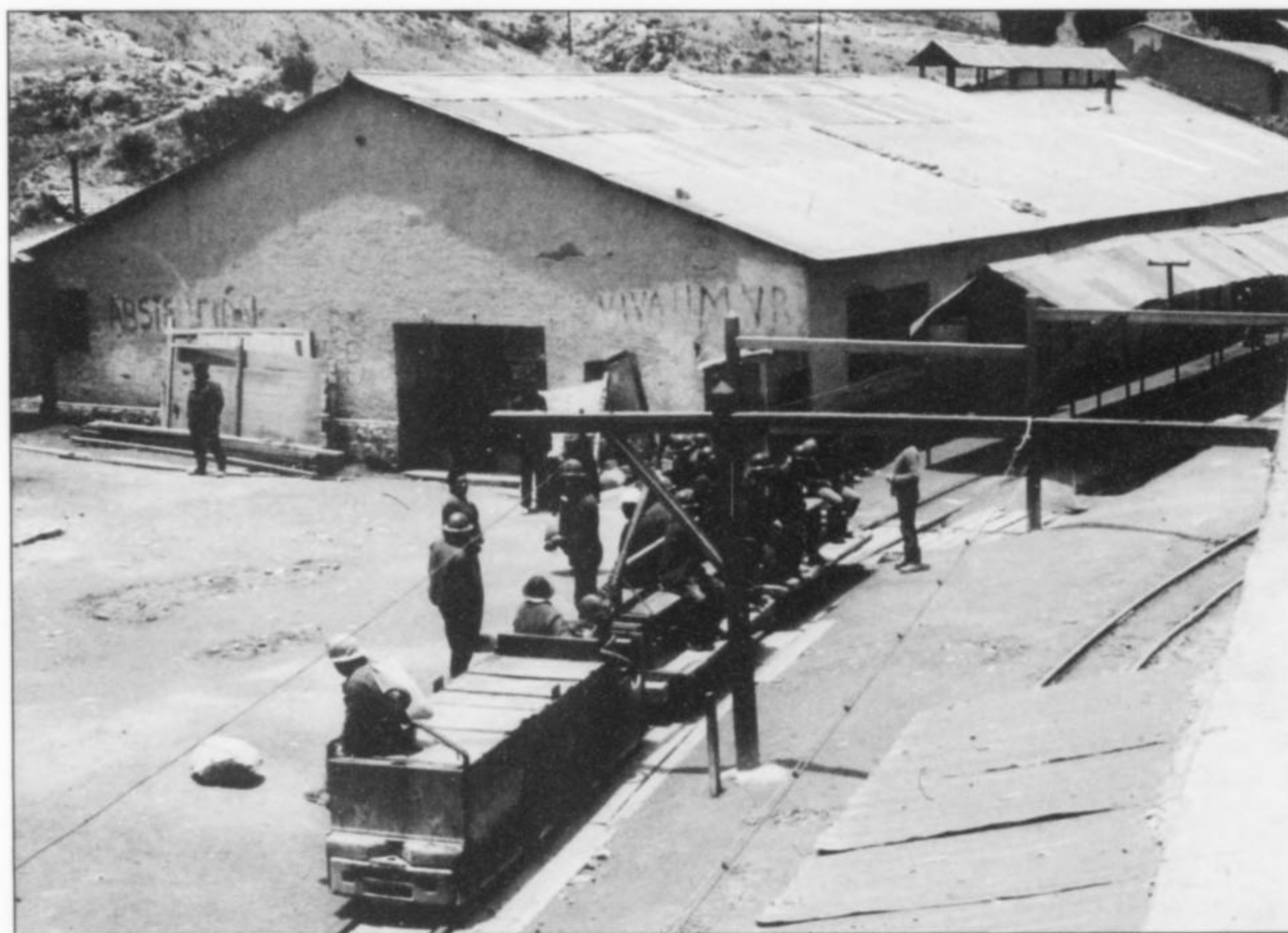
Figure 13. Mine train at the portal of the Siglo XX Tunnel, 1975. Rock Currier photo.
