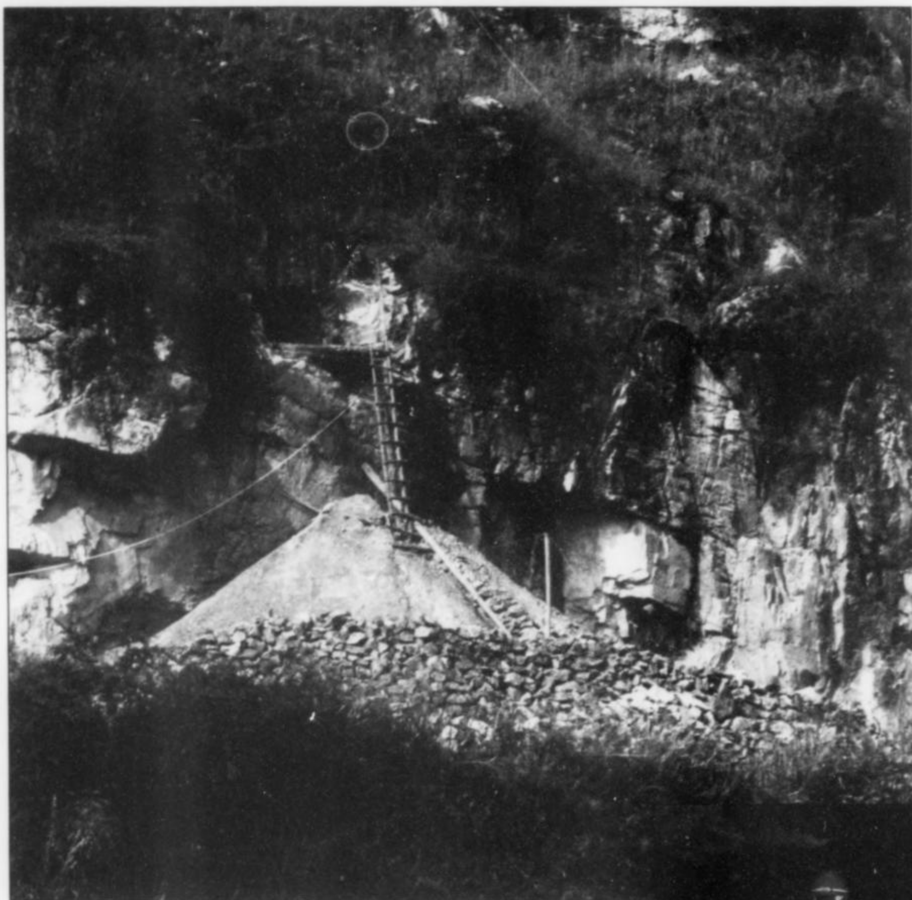
Figure 5. Exploratory tunnels have been driven into the hillside using the most primitive methods. Ottens photo.
