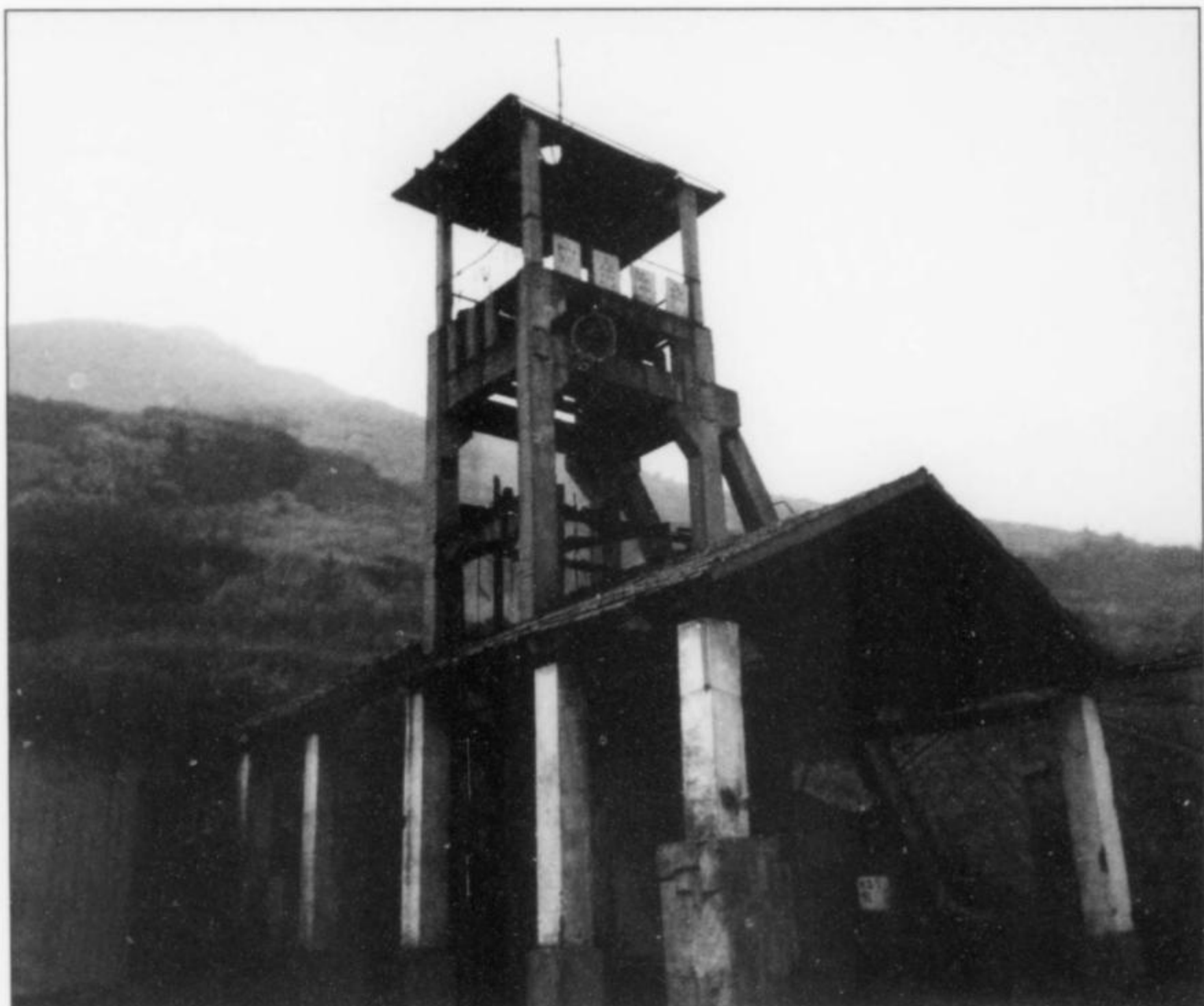
Figure 1. Old headframe of the Fengjiashan I shaft. Weigang Chen photo.
