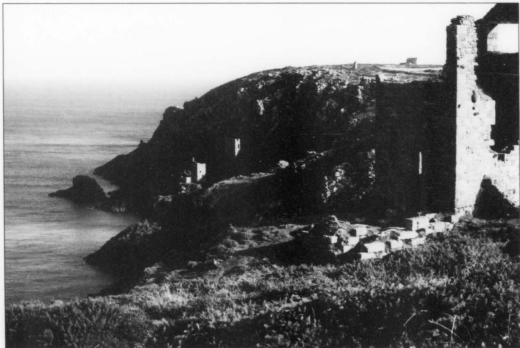
Figure 5. One of the World's most photographed scenic spots—"the Crowns" engine houses of the Botallack mine. The upper house held the hoisting engine, and the lower, the pumping engine for an inclined shaft that ran 414 meters (1,360 feet) under the sea. It cannot be seen from this angle, but there is a vertical cliff on the far side of the upper house.
