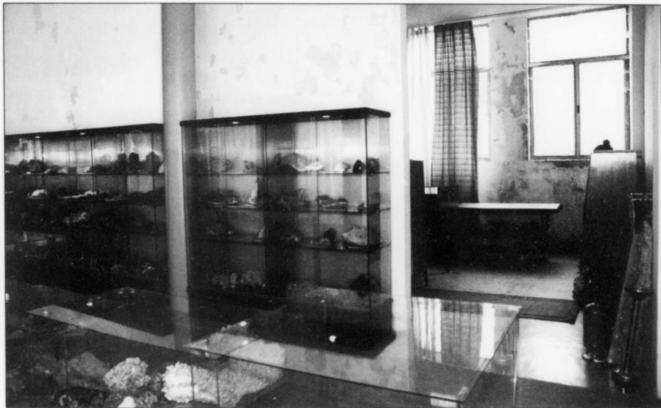
Figure 60. Interior of the Trepča museum building, showing signs of deterioration. B. Larderet photo.
