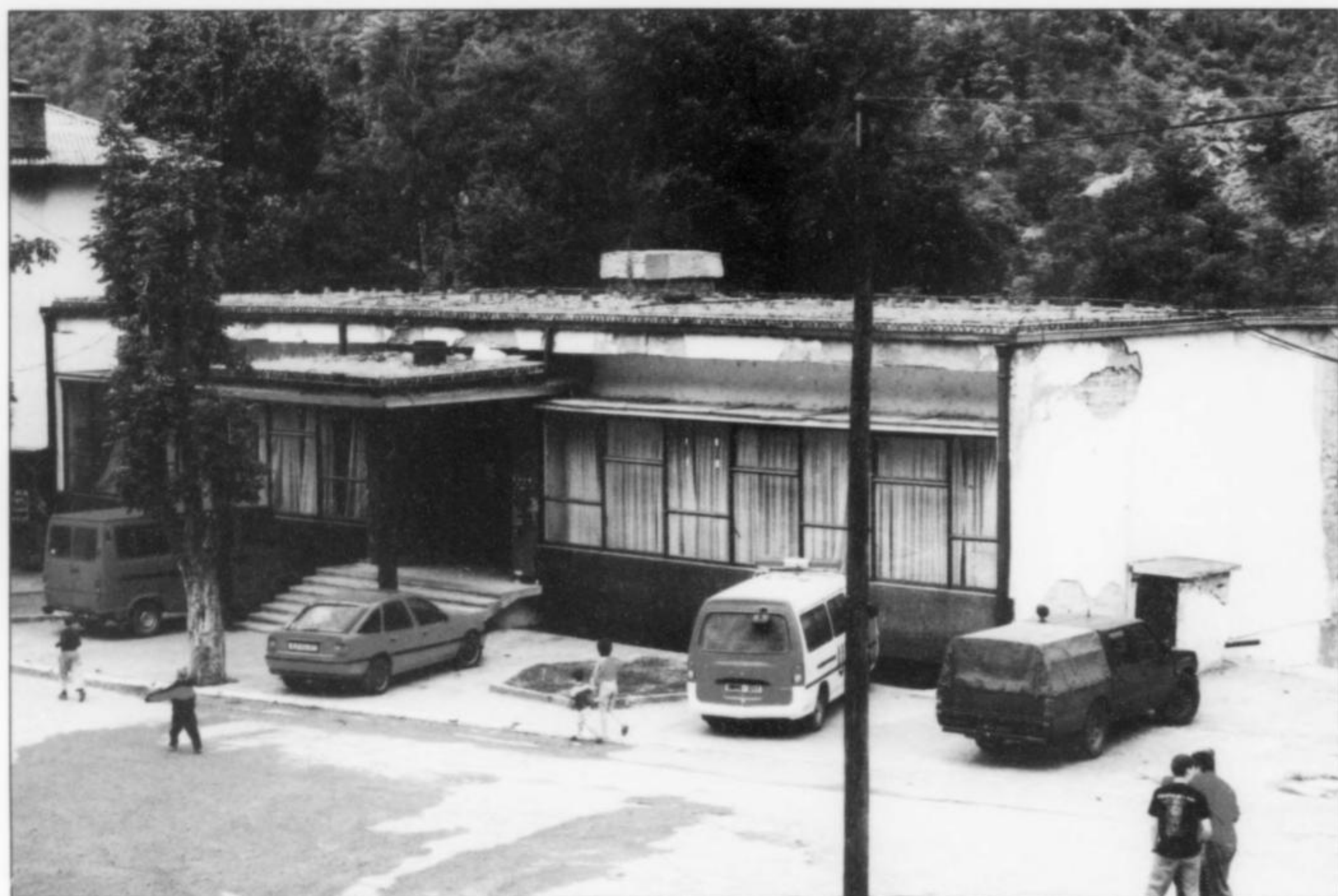
Figure 59. The Trepča museum building, showing signs of deterioration. J. Balazuc photo.
