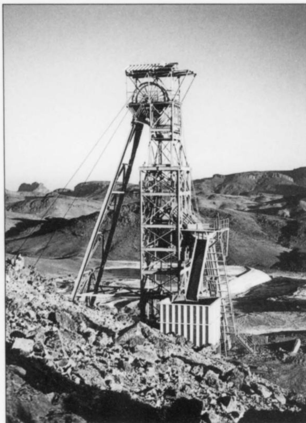
Figure 10. Landmark: Shaft 3 at Bou Azzer. Behind it, mud tanks for ore preparation. May 2001. Georges Favreau photo.
