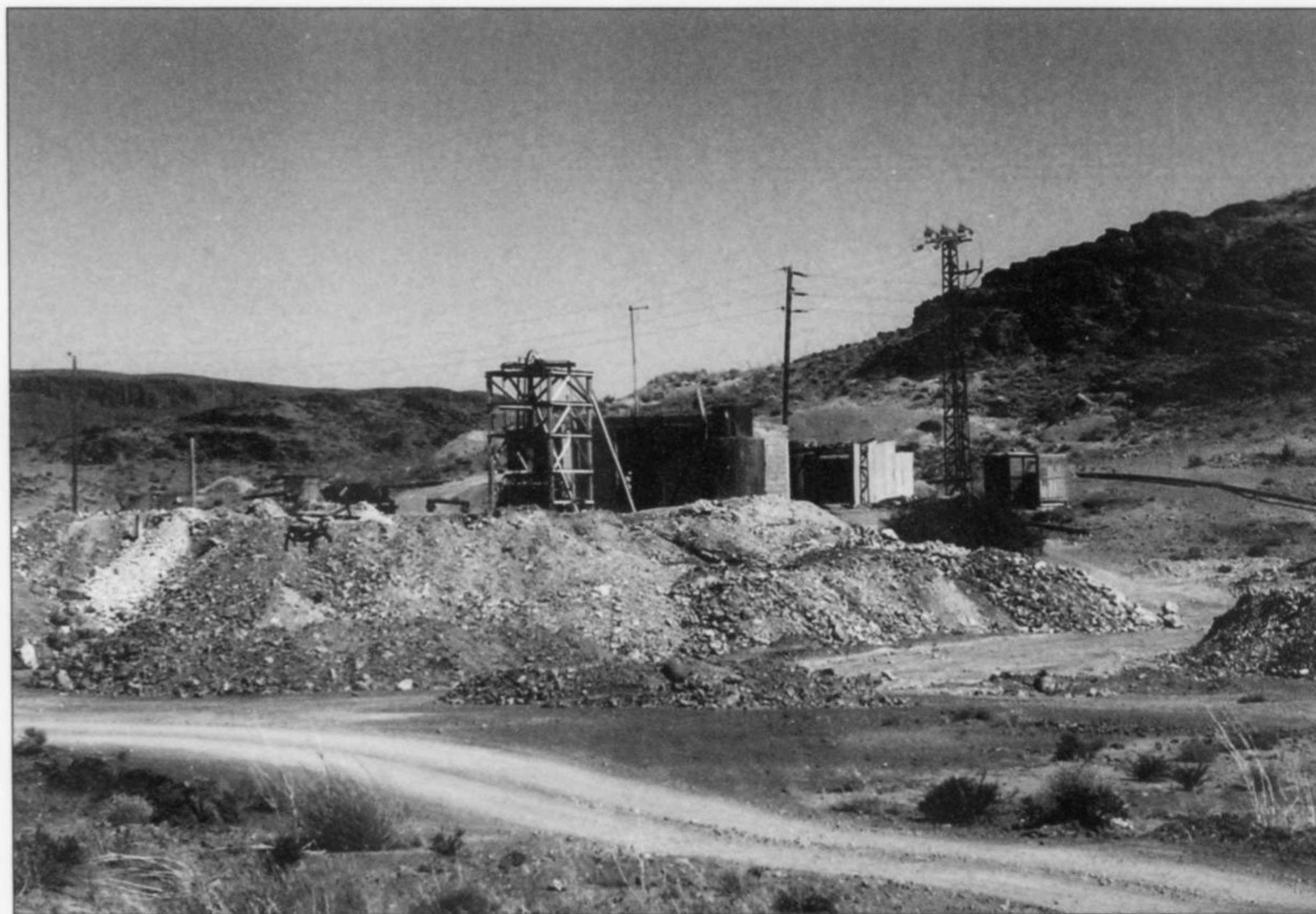
Figure 20. Shaft at Oumlil Center, April 2004. Georges Favreau photo.
