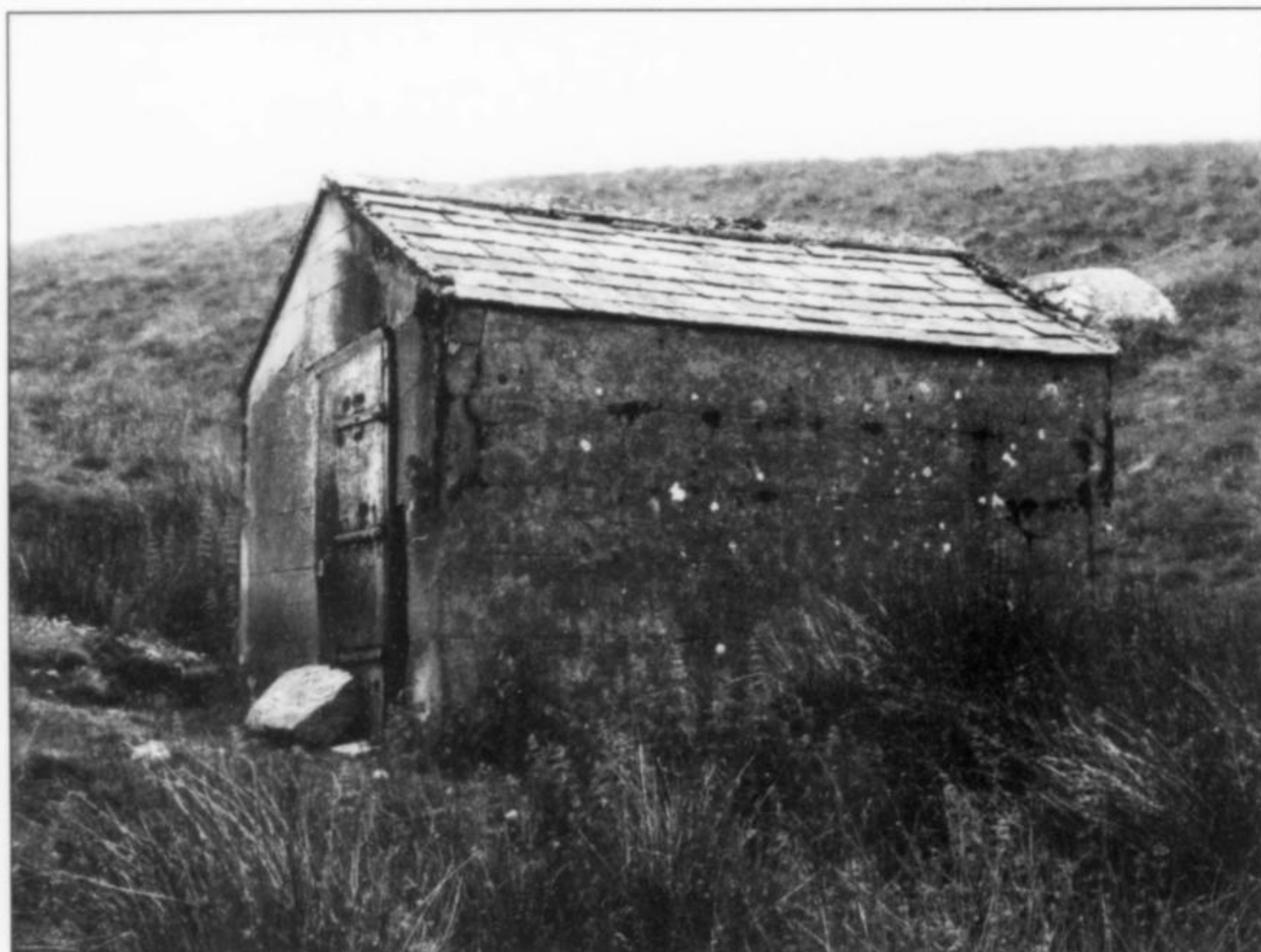
Potts Gill mine, an old stone or concrete shed with an iron door (possibly a powder magazine).
