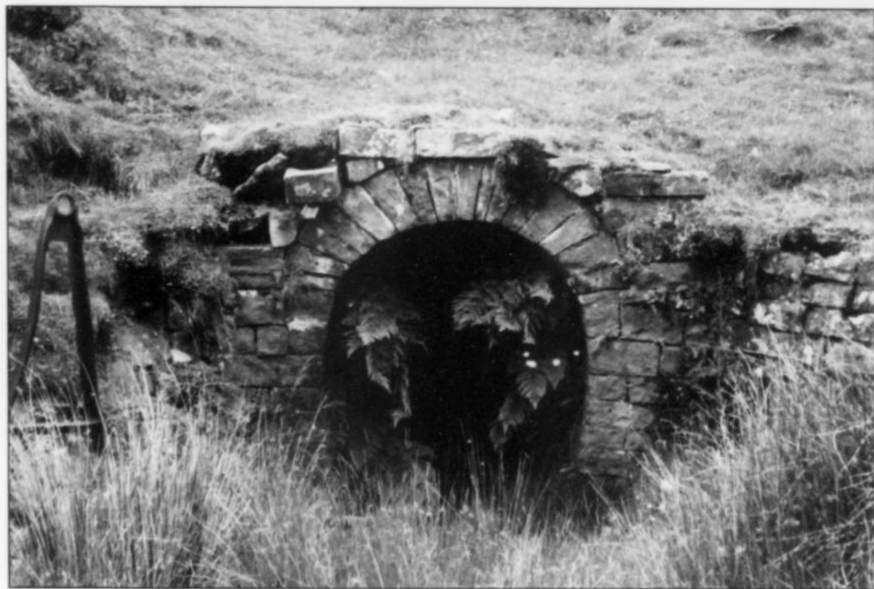
(Left) Stone-arched portal to the Middle level of the Greenlaws mine. Jesse Fisher photo (2005).
