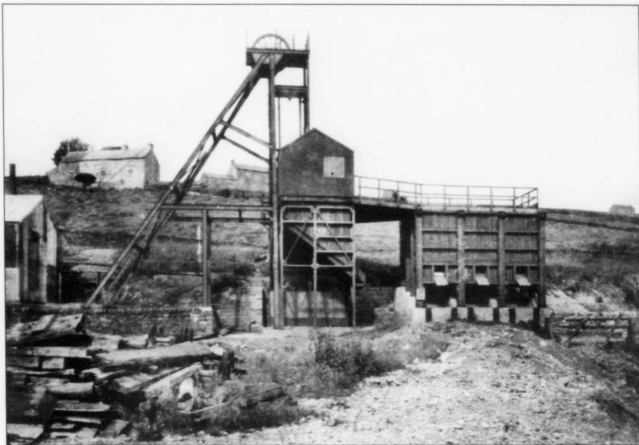
Headframe and ore bins at the St. Peter's mine near Spartlea, East Allendale (early 1900s). Beamish Museum photo archives.
