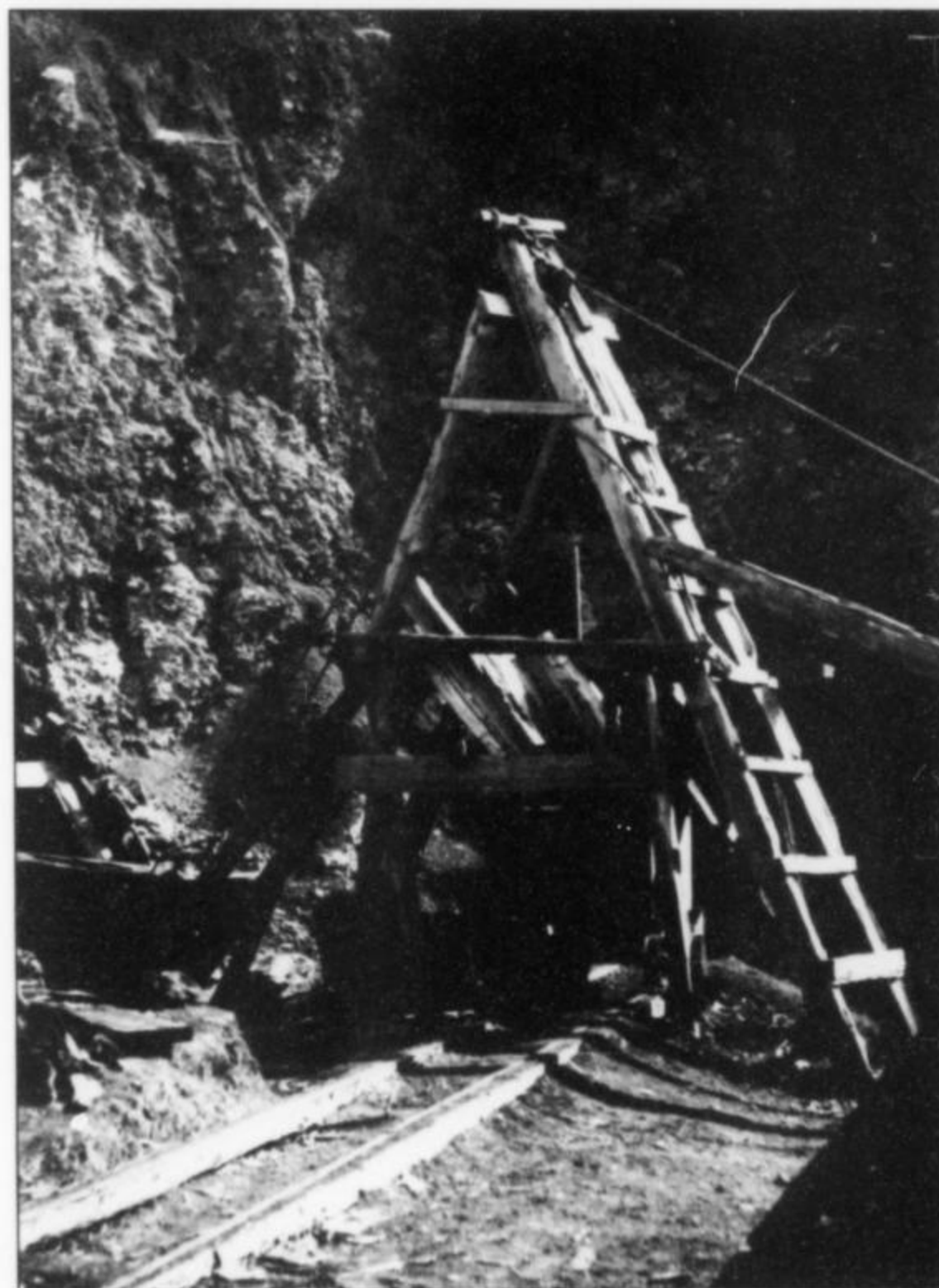
Figure 12. Headframe for one of the two 16-meter inclined shafts at the Dallas mine. (Courtesy Collector's Edge Minerals .)
