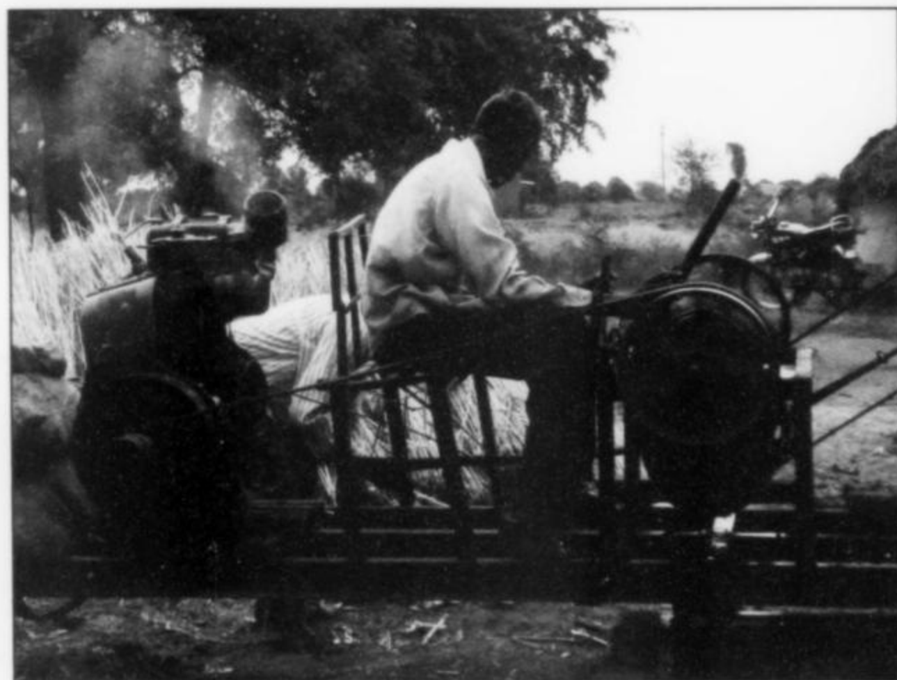
Figure 2. The hoisting engine for lowering people and supplies down into the well, and raising specimens out.
