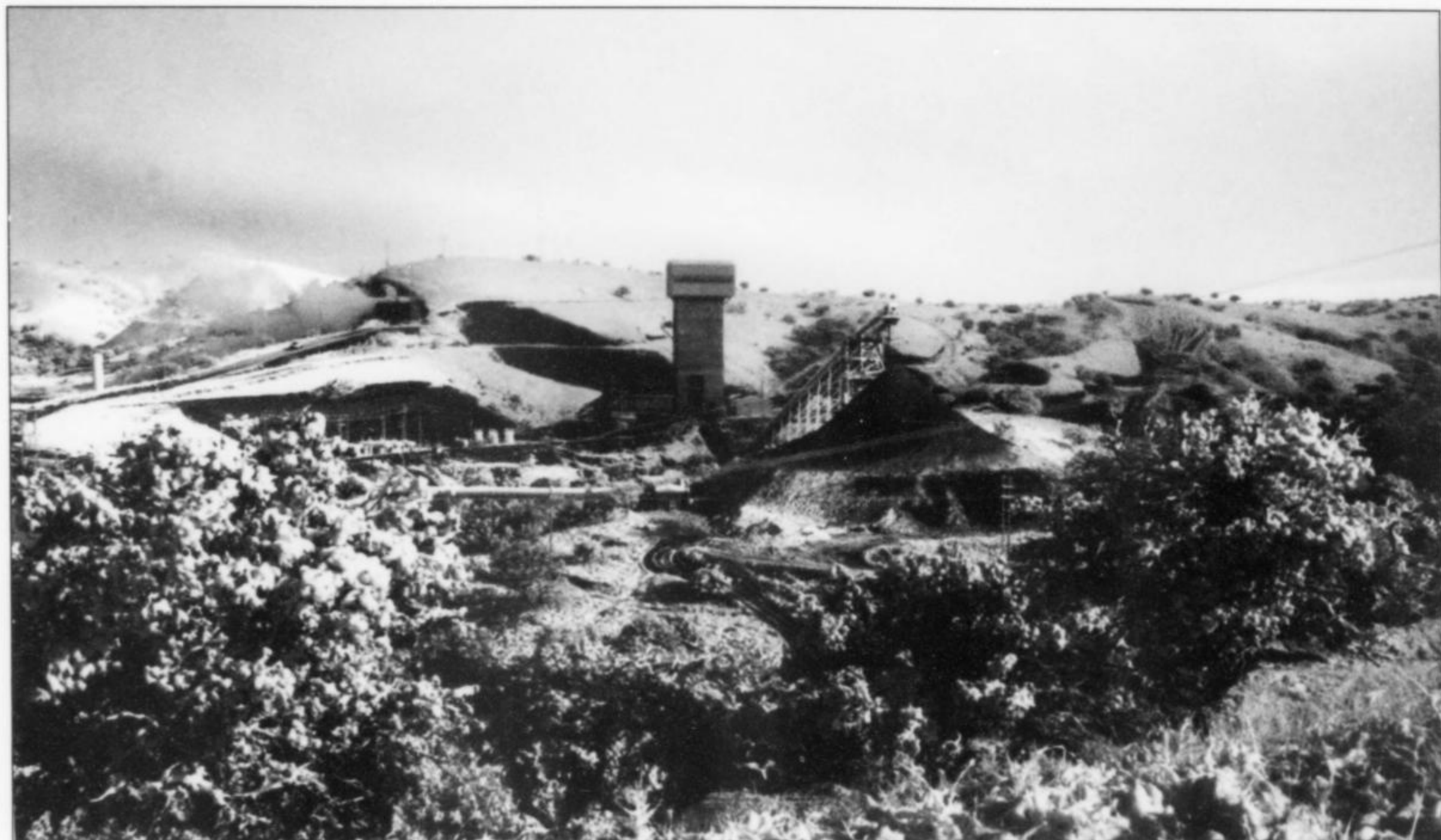
Figure 2. The Milpillas mine site (photo courtesy of Salvador Ortiz and Francisco Quintana, Peñoles Company).
