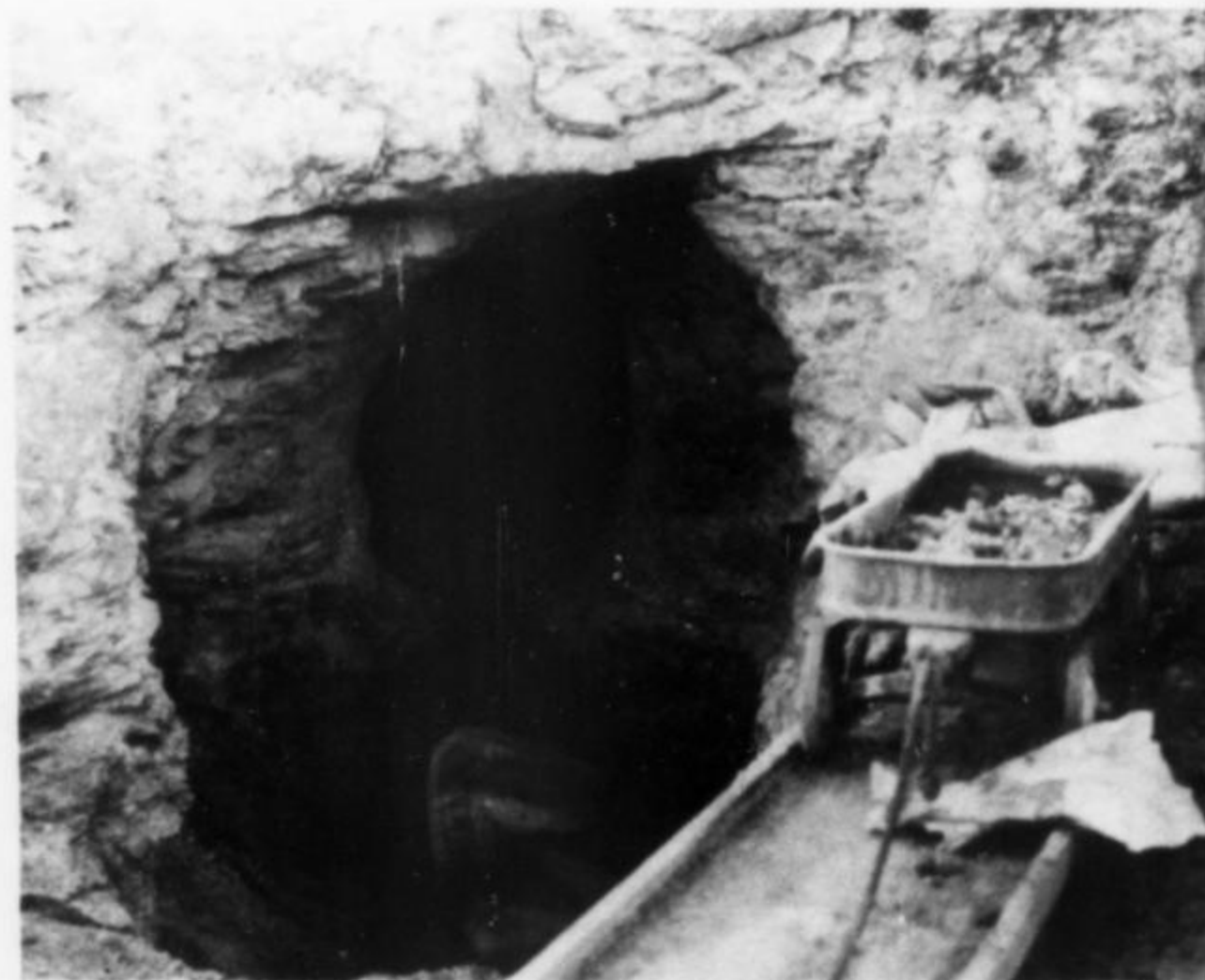
The succession of pockets that produced the large quantity of tourmaline at Plumbago Mountain, Maine in 1972. The contents of the pockets were placed in the toy wagon which was then pulled up the ramp to a dump where it was rough-sorted and sacked or boxed.
