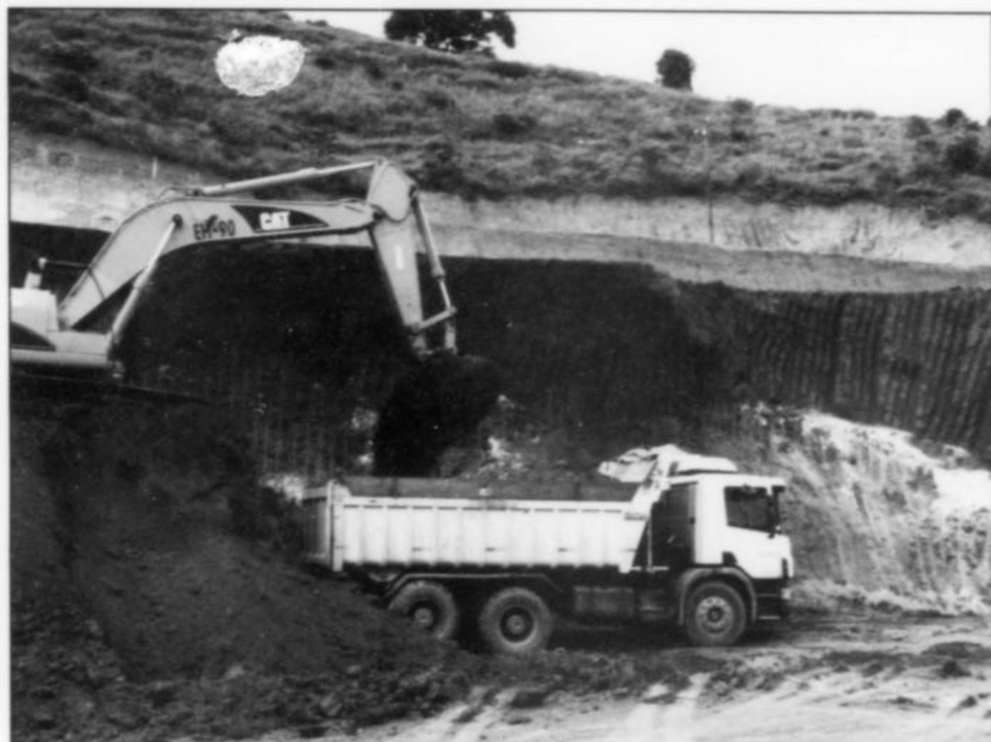
Figure 15. Excavation of emerald-bearing laterite at the Belmont mine. Guido Steger photo, 2006.
