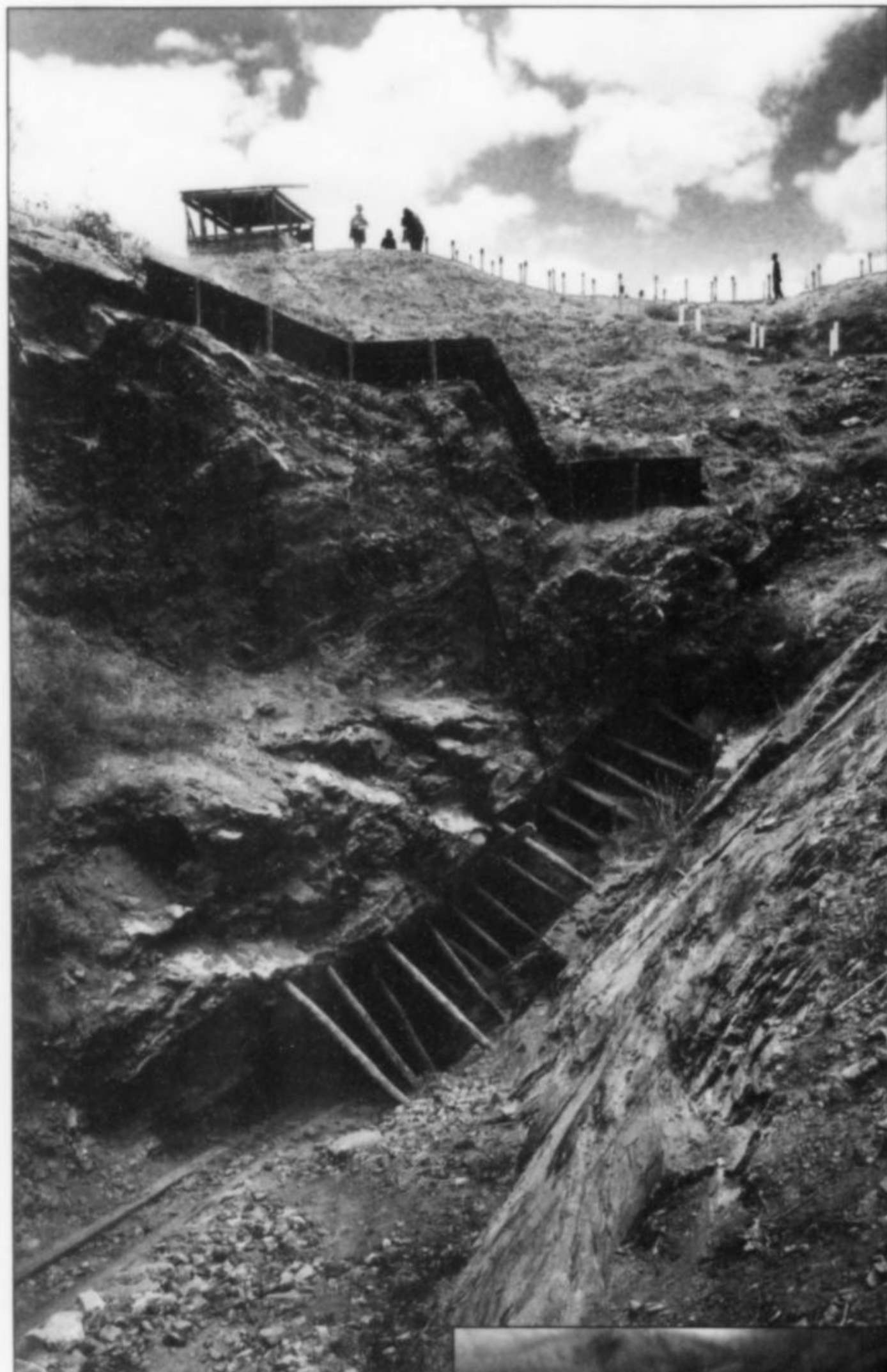
Figure 31. Old open cut and entrances to underground workings at the Samax mine in Merelani Block A. Anthony Kampf photo, 1995.
