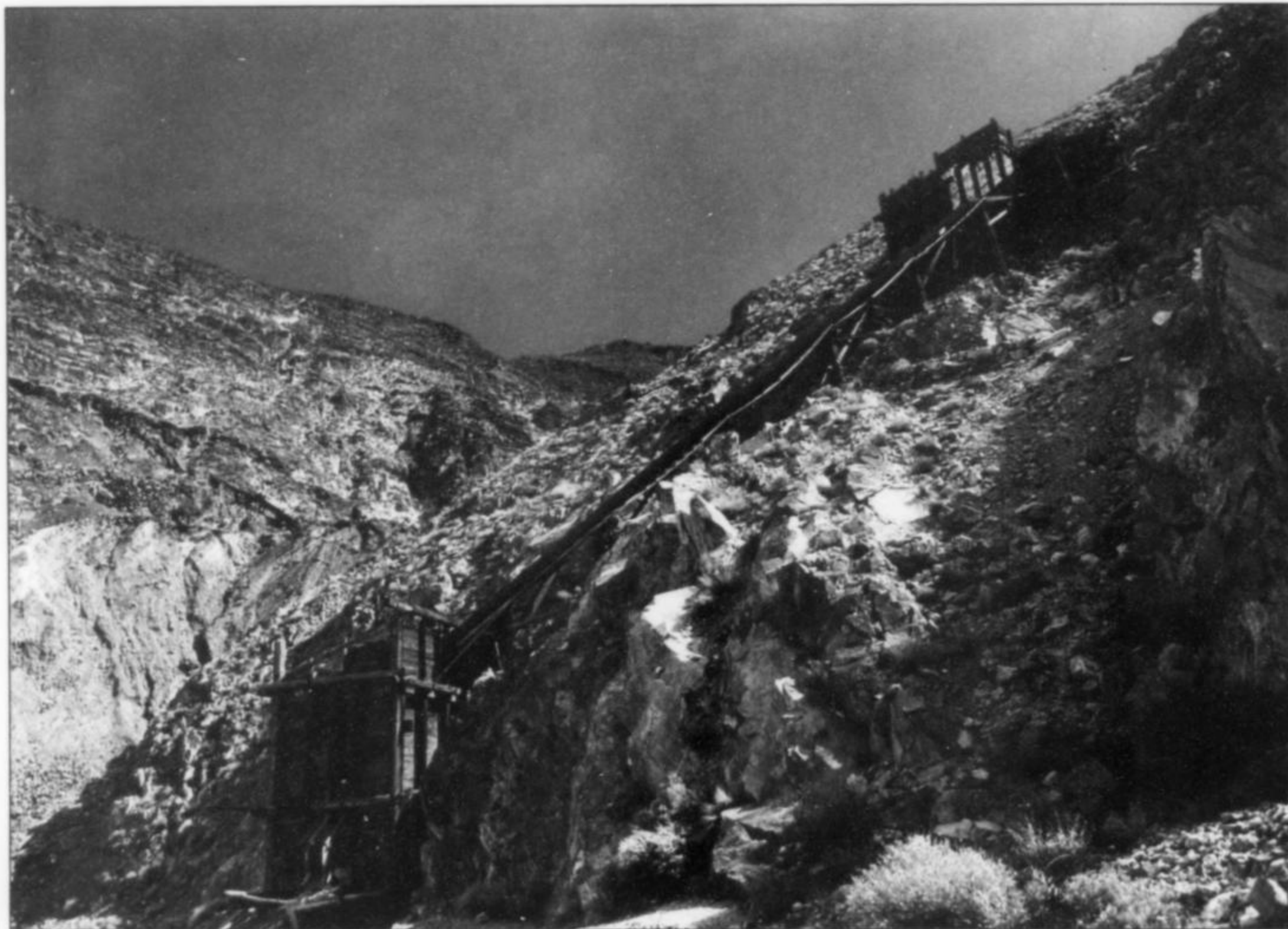
Figure 6. Ore chute just below the level of the Brown Monster mine entrance.
