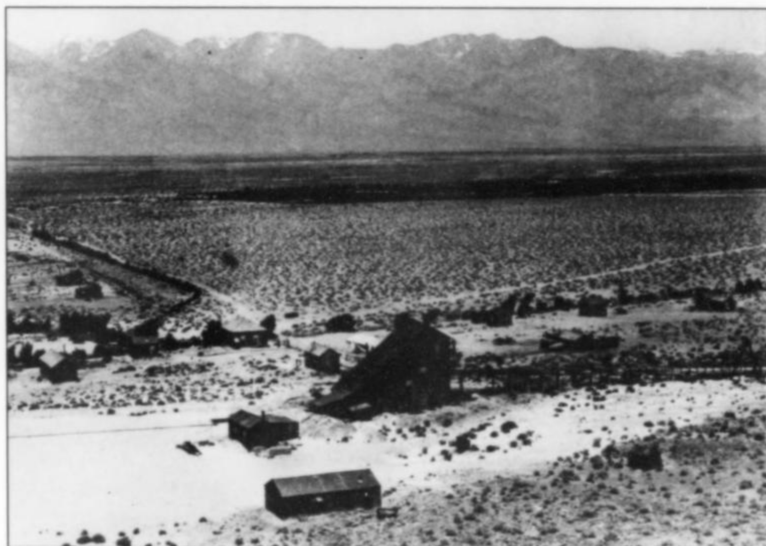
Figure 2. Reward mill and other buildings, ca. 1890.
