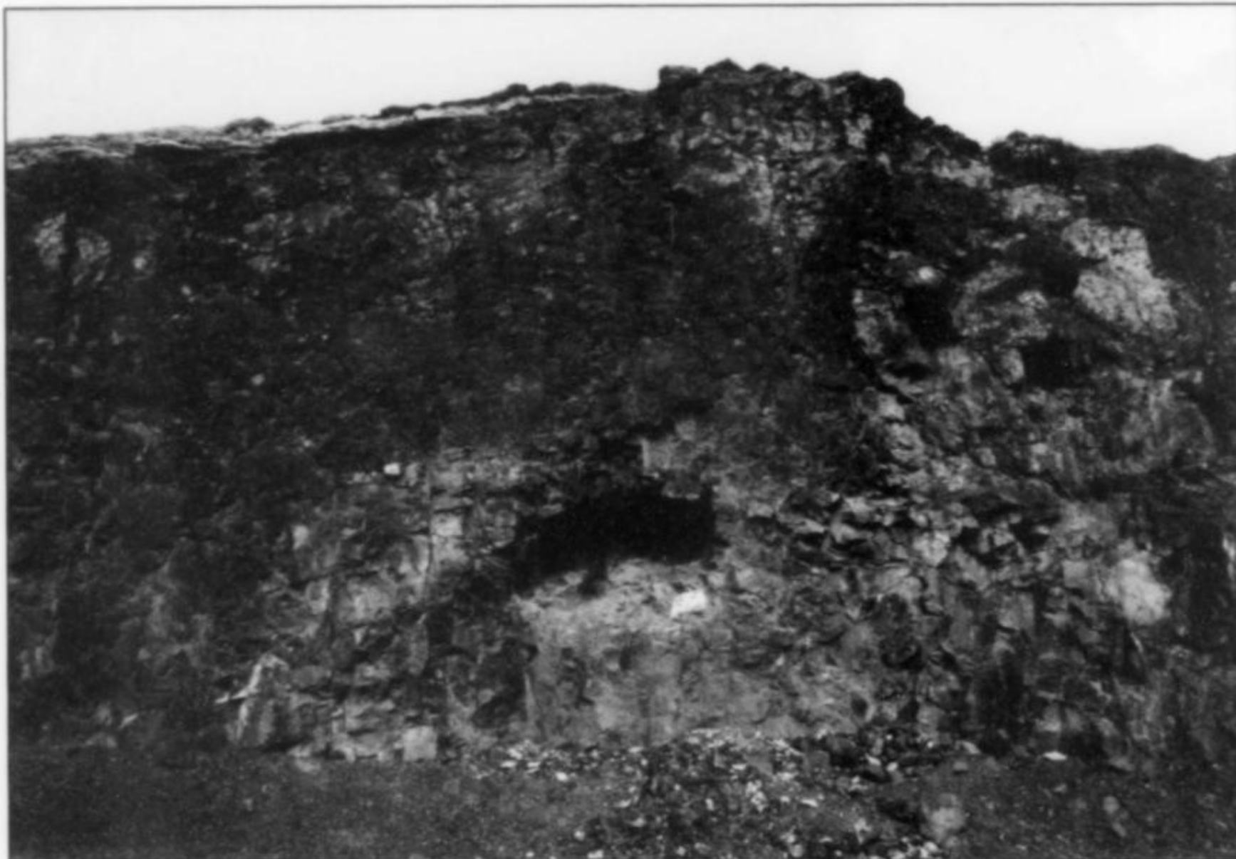
Figure 4. Excavation in a mineralized diapir of the lower colonnade of the Orange Mountain second flow. Mark Bianchi photo, 2008.
