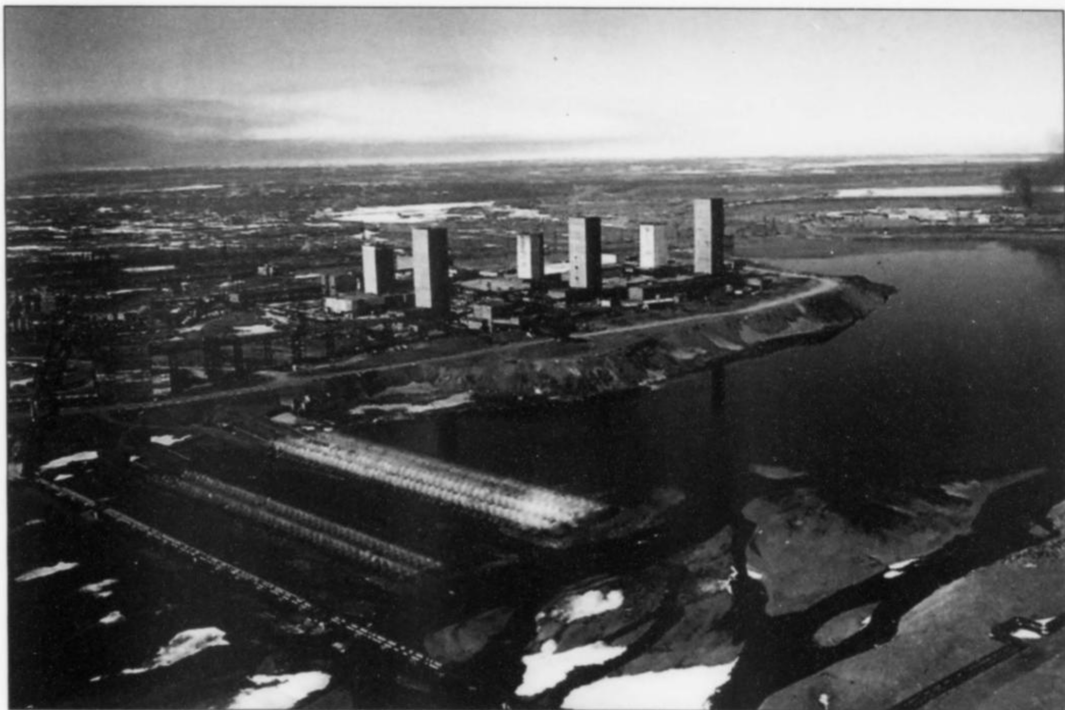
Figure 2. Aerial view of the Talnakh mining complex on the east bank of the Kharaelakh River. The six square towers are headframe structures over Oktyabr mine shafts.
